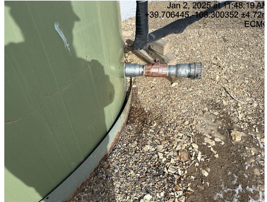
Staining from under tank
