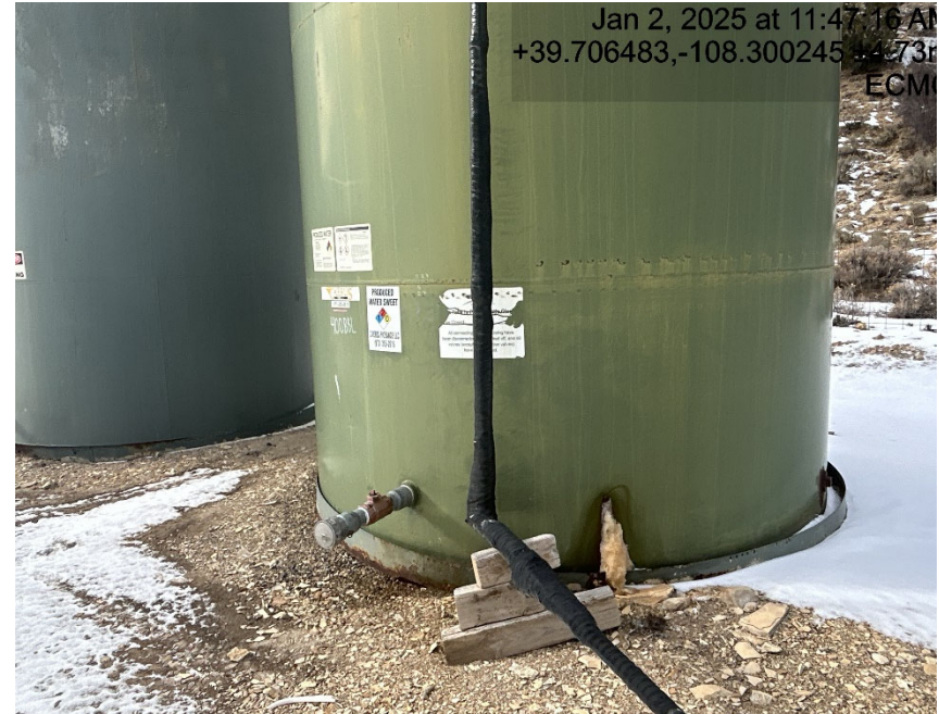
Tank leaking
