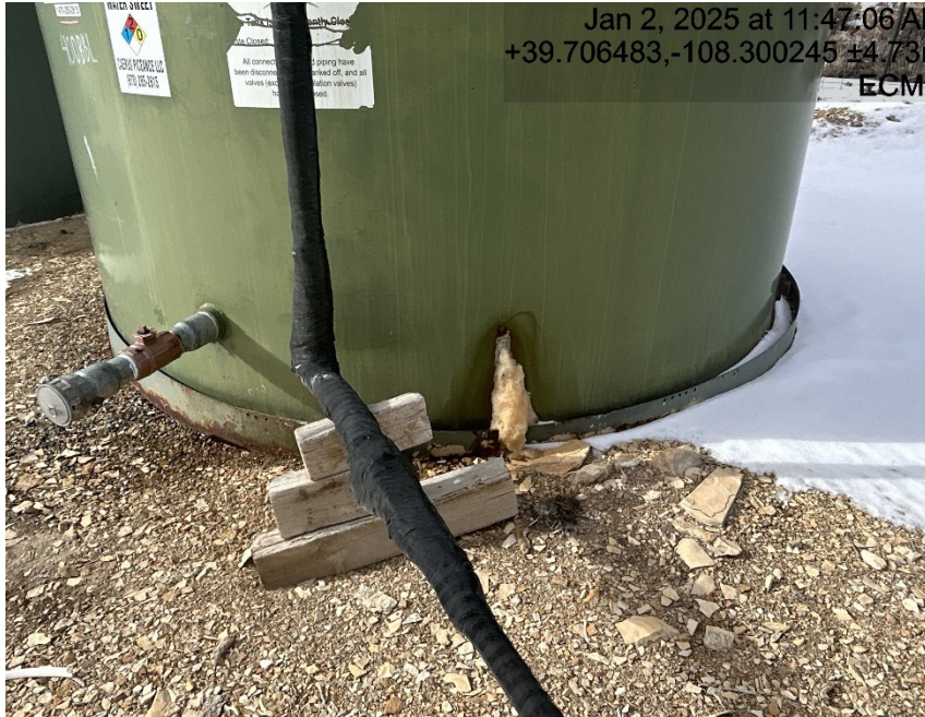
Tank leaking
