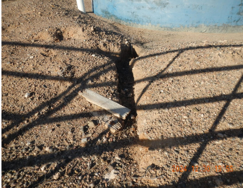
5. Erosion channel in SW corner of tank berm.
