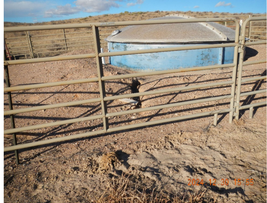
6. Additional view of erosion channel in SW corner of tank berm.
