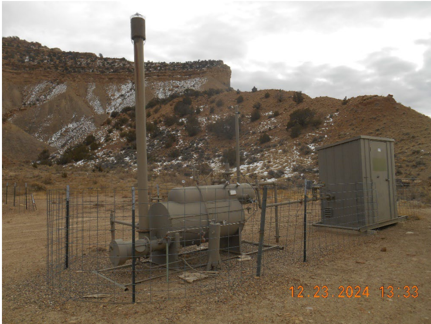
Separator and Meter housing
