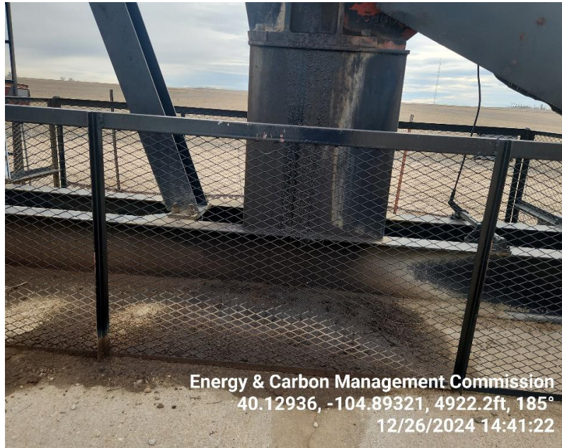
Photo 5 Stained concrete & soil on both sides of the pump jack.
