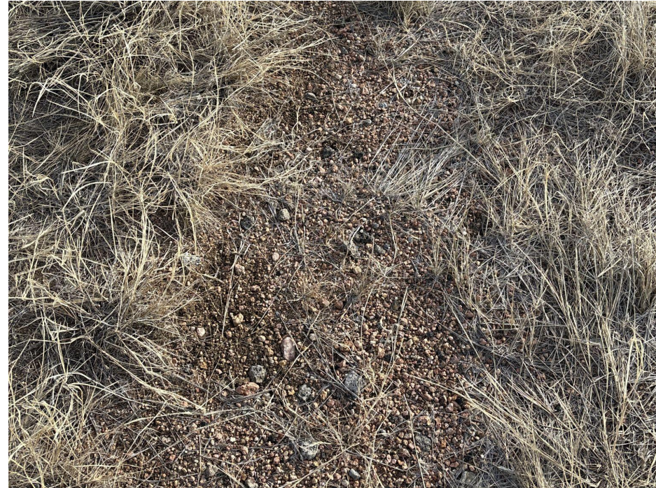
Photo 2. Gravel/road base remains along entire length of access road.
