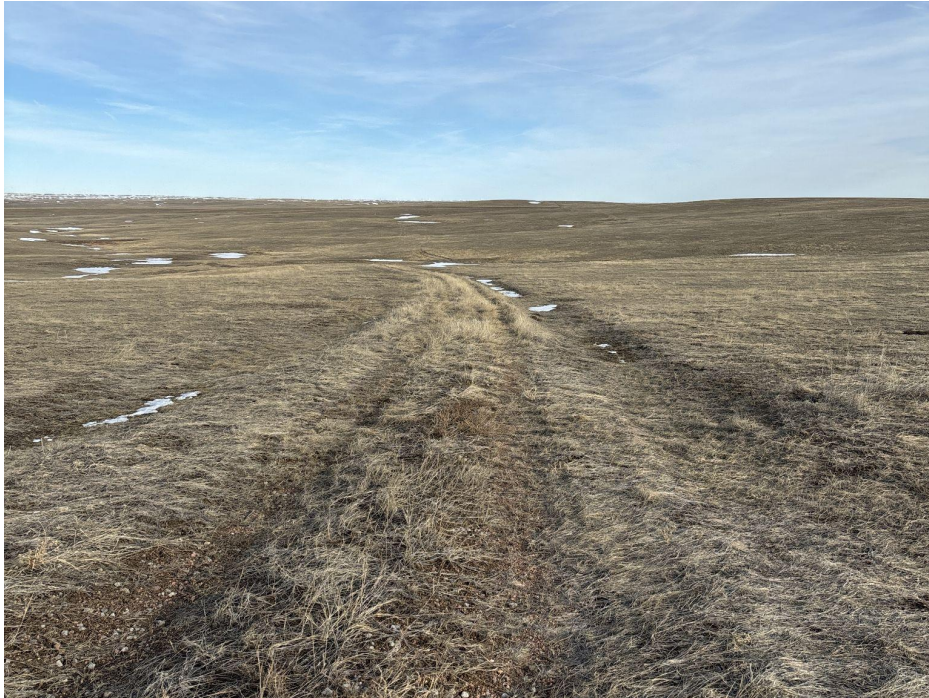
Photo 1. Photo taken Looking east along access road. Access road does not appear to have been recontoured or reclaimed. Gravel has not been removed.
