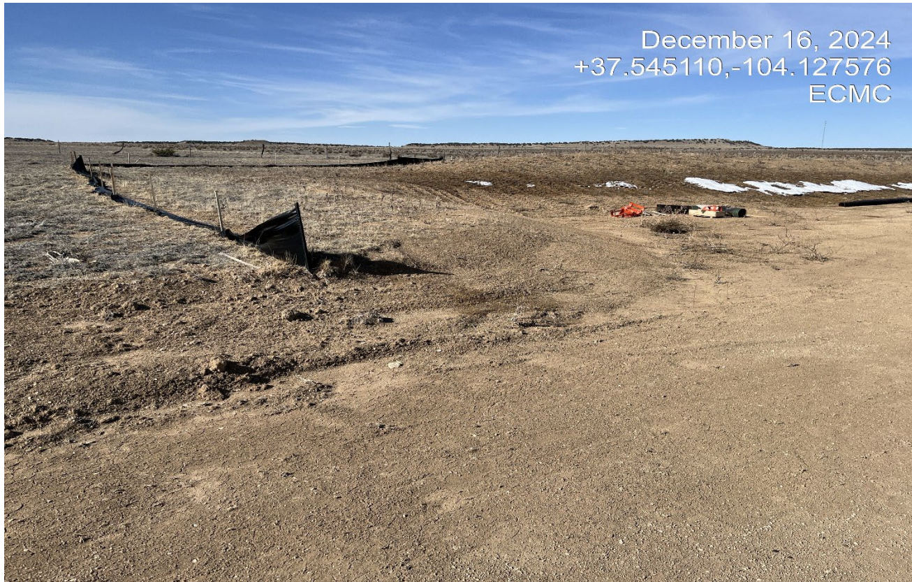
Photo 4. Facing southwest at the location. The silt fence is not maintained. Unused equipment and pipe have not been removed.
