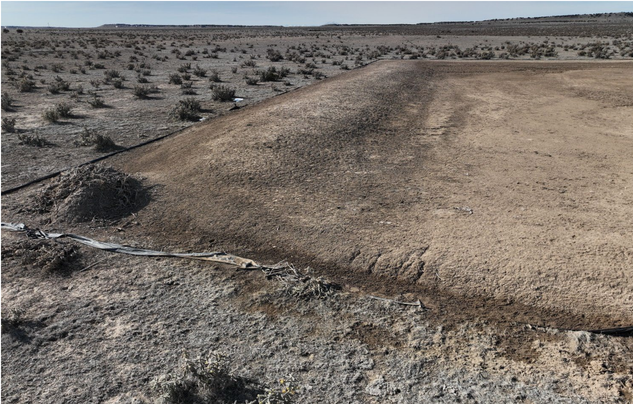
Photo 4. Southeast corner of the location facing southwest. The silt fence is down and not maintained. The pile of debris in the corner has not been removed.
