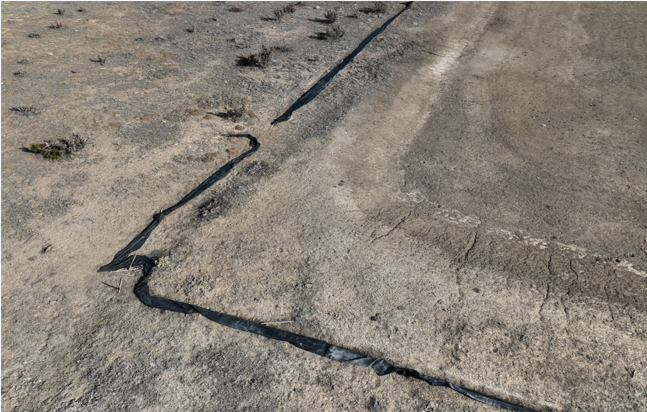
Photo 7. Facing down toward the northwest corner showing the silt fence is not maintained and there is erosion riling along the cut slope.
