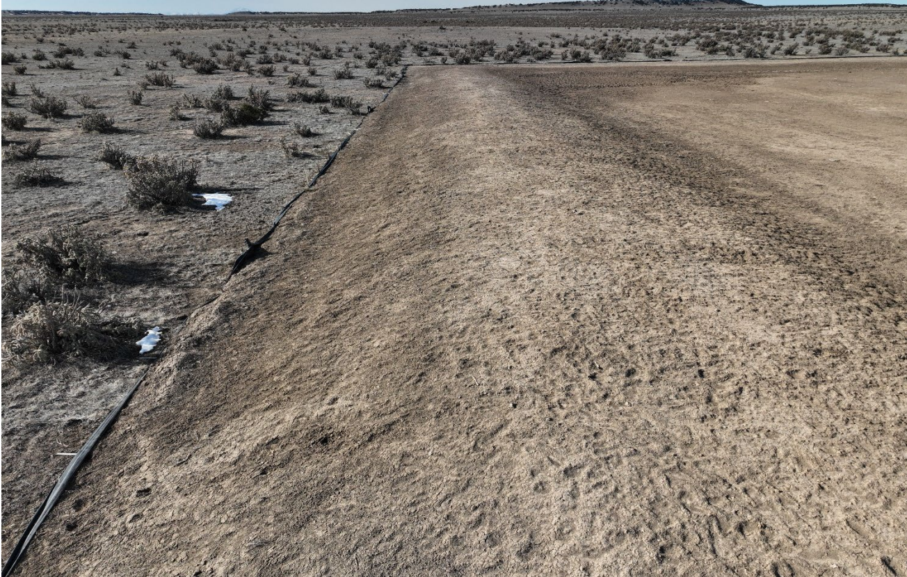
Photo 5. Facing toward the soil stock pile. The topsoil has not been seeded and stabilized and the silt fence is in disrepair.
