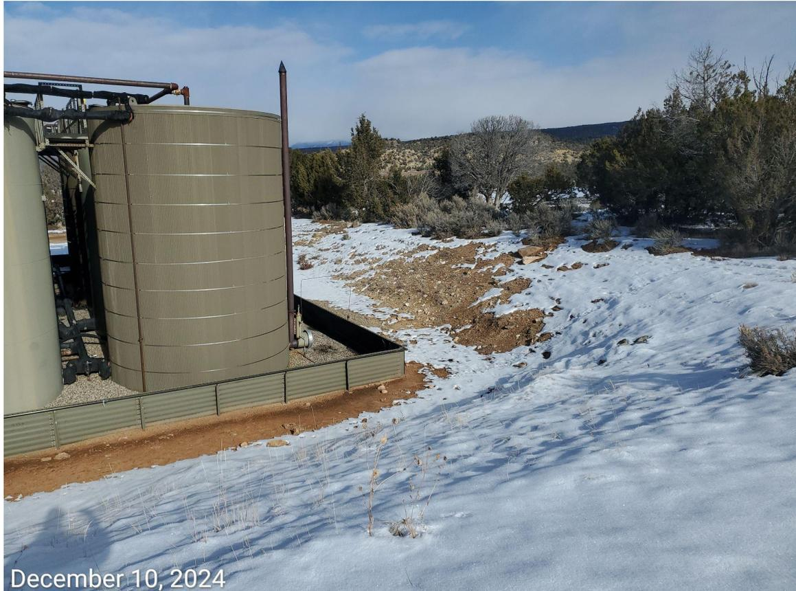
**Photo 3:** Photos taken from the interim areas of the battery facility. Limited inspection due to snow cover. Unable to find evidence within areas that were observable, that additional reclamation work has been performed, and BMPs to stabilize the seeded soils implemented. No resolution has been submitted stating work was performed.
