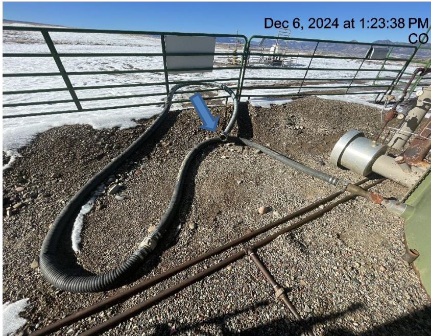
Photo # 2706 Open ended load line
