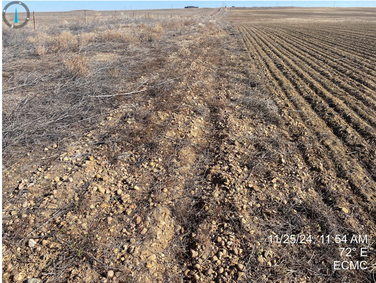
Photo 4. Taken from the approximate midpoint of the access road, facing east. Photo illustrates road base material remains on the access road, which does not appear to have been reclaimed.
