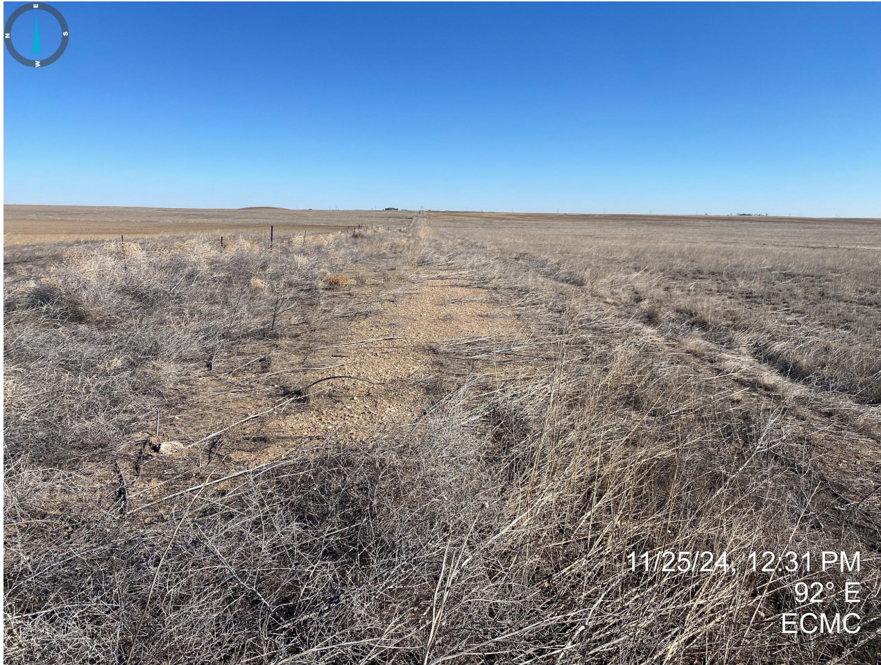
Photo 6. Taken from the access road north of the location, facing east. Photo illustrates road base material remains on the access road, which does not appear to have been reclaimed.
