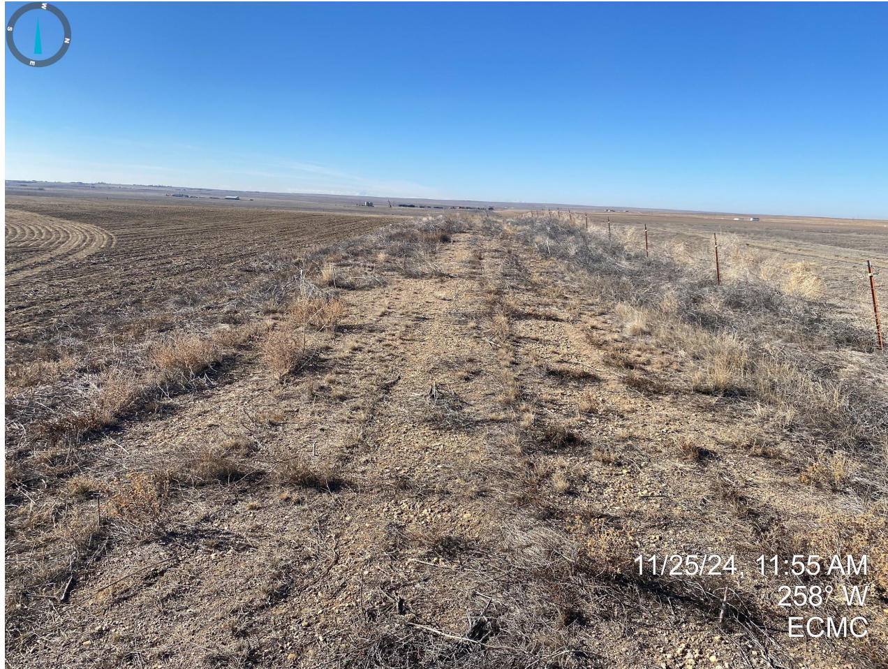
Photo 5. Taken from the approximate midpoint of the access road, facing west. Photo illustrates road base material remains on the access road, which does not appear to have been reclaimed.
