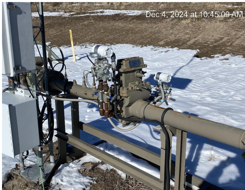
No visible display of gas meter calibration
