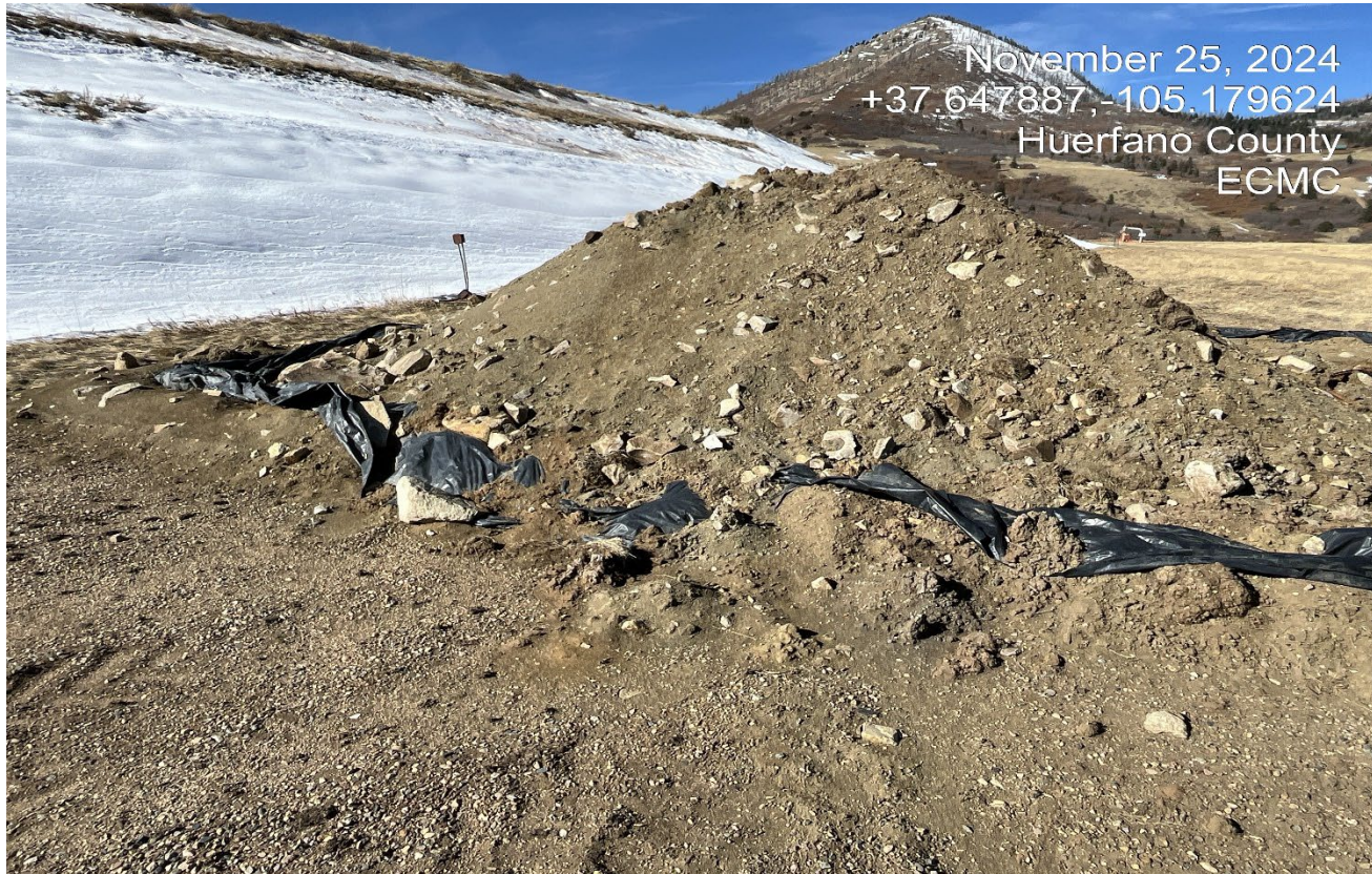
Photo 2. There is a material pile stored from the excavated pit. The berm around the pile is inadequate and material has fallen outside of the containment.
