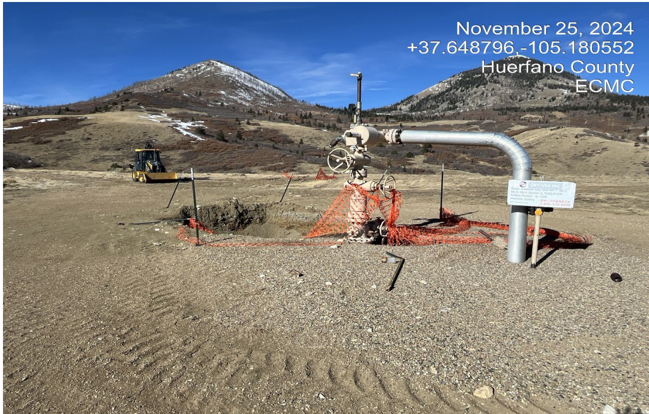
Photo 5. The orange fence is displaced around the excavated area near the well. .
