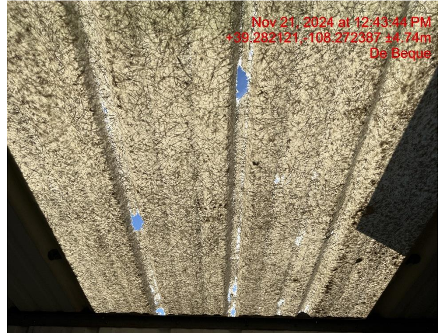
Photo # 9557 Gas meter building roof paneling is damaged/wildlife hazard available for entry by wildlife
