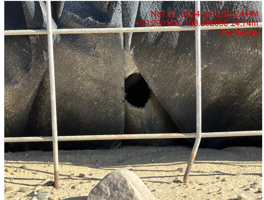
Photo # 9516 Multiple holes and tears in secondary containment liner/liner needs maintenance also the liner is deteriorating and lacks integrity
