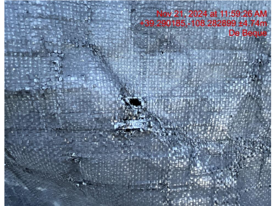
Photo # 9511 Multiple holes and tears in secondary containment liner/liner needs maintenance also the liner is deteriorating and lacks integrity
