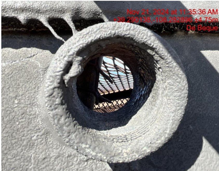
Photo # 9501 Tank port open to wildlife/wildlife hazard/ available for entry by wildlife
