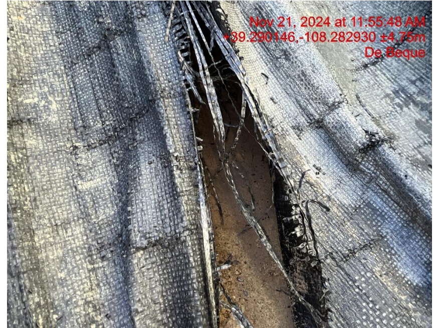
Photo # 9507 Multiple holes and tears in secondary containment liner/liner needs maintenance also the liner is deteriorating and lacks integrity
