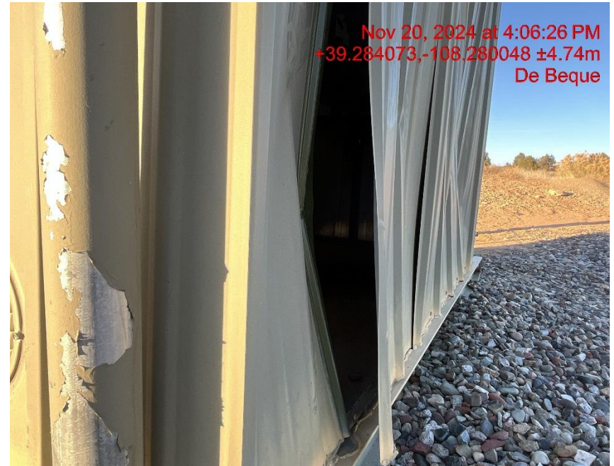
Photo # 9467 Gas meter building/siding is damaged/wildlife hazard available for entry by wildlife
