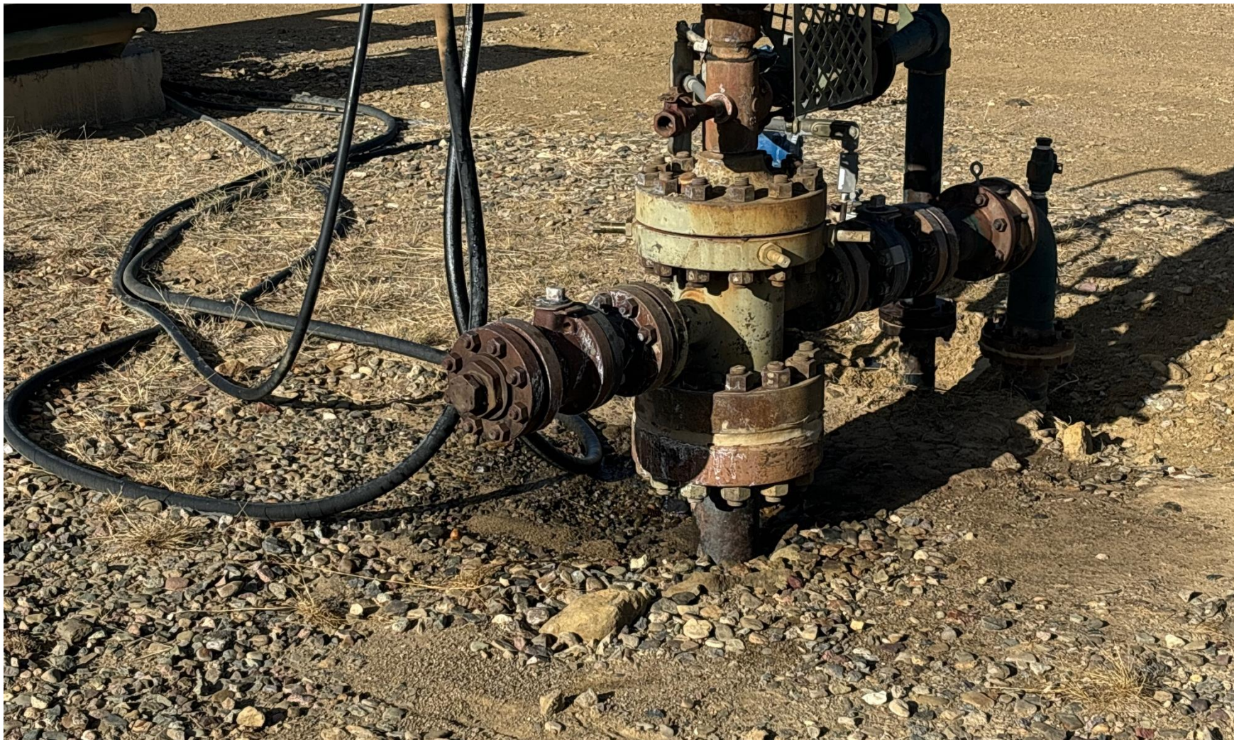
PHOTO 4: AREA OF IMPACTED SOIL AROUND WELLHEAD APPEARS TO BE FROM LEAKING DRIVEHEAD. Conduct maintenance on equipment, cleanup stained material and review self inspection processes. COMPLY WITH RULE 1002,(2).D. CA DATE 12/1/2024.
