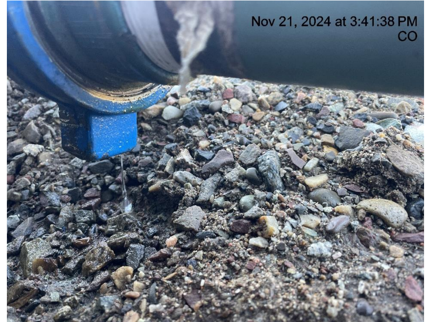
Photo # 963 Mechanical Condition – possible dump line leak
