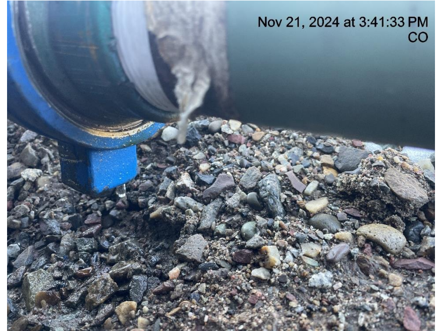
Photo # 961 Mechanical Condition – possible dump line leak
