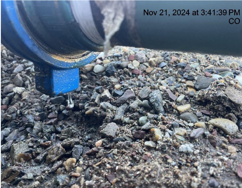
Photo # 964 Mechanical Condition – possible dump line leak
