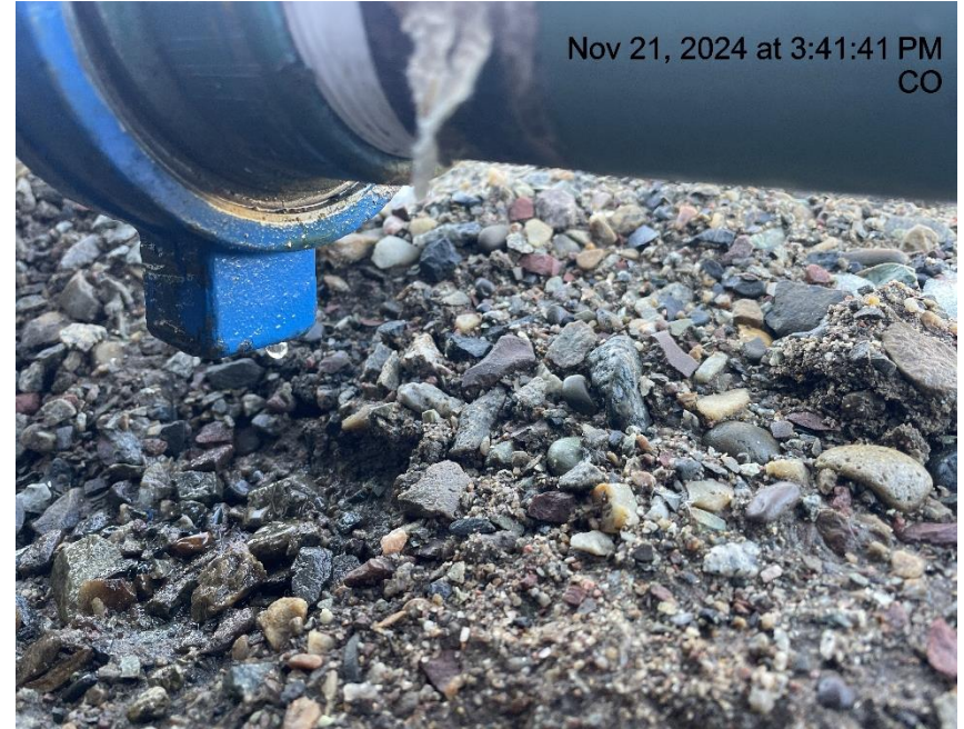
Photo # 965 Mechanical Condition – possible dump line leak
