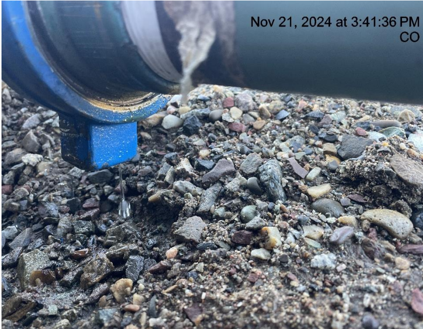
Photo # 962 Mechanical Condition – possible dump line leak
