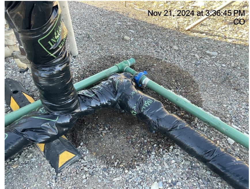
Photo # 959 Mechanical Condition – possible dump line leak
