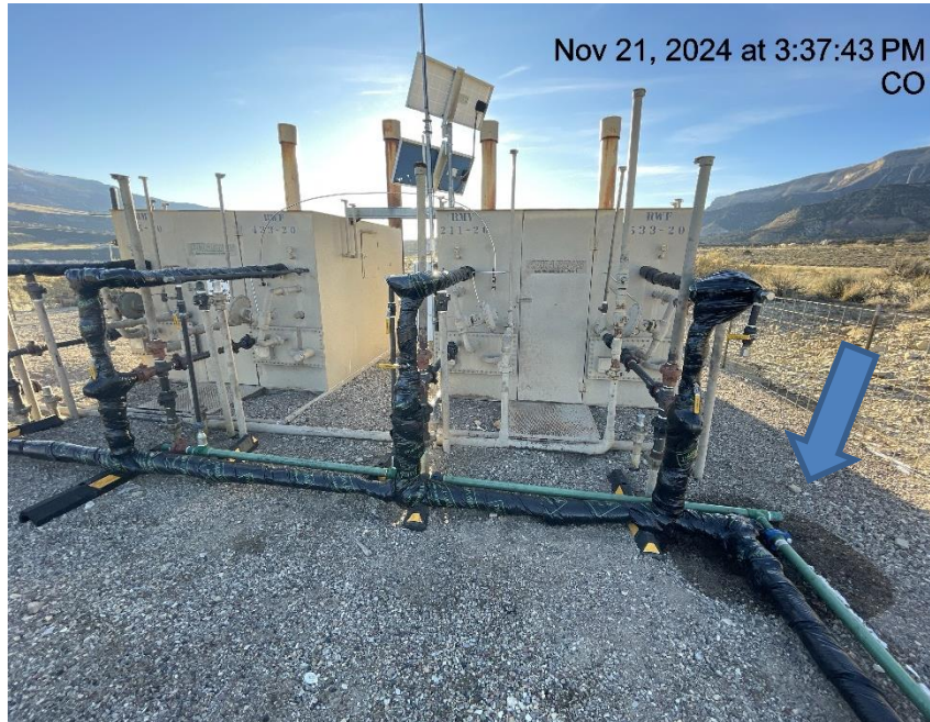
Photo # 958 Mechanical Condition – possible dump line leak
