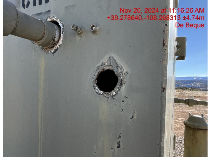
Photo # 9275 Open hole on separator building/wildlife hazard available for entry by wildlife
