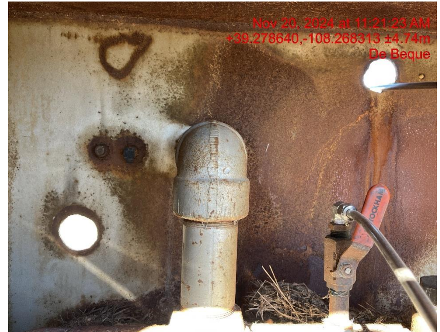
Photo # 9279 Open holes on separator building/wildlife hazard available for entry by wildlife
