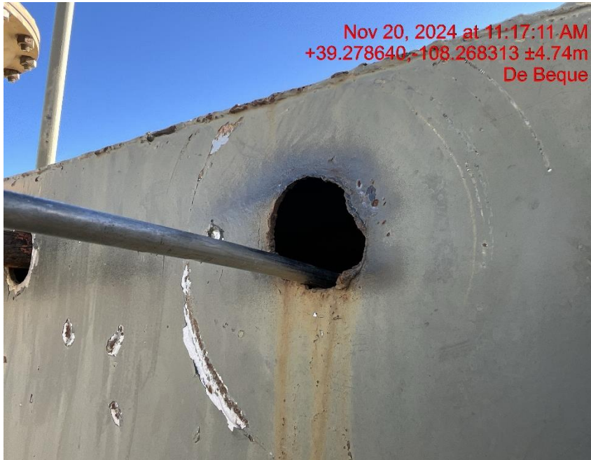
Photo # 9278 Open hole on separator building/wildlife hazard available for entry by wildlife
