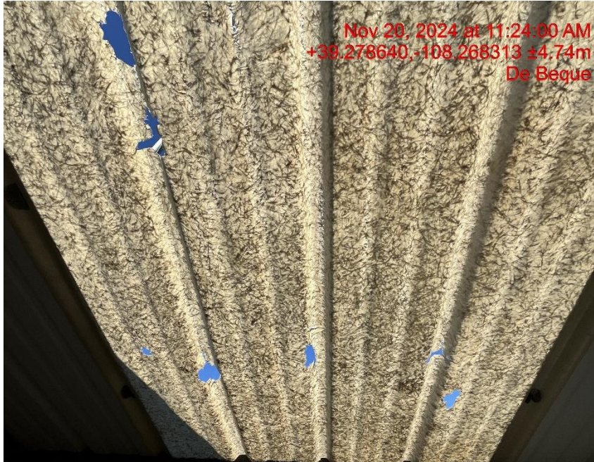
Photo # 9282 Gas meter building roof paneling damaged/wildlife hazard available for entry by wildlife
