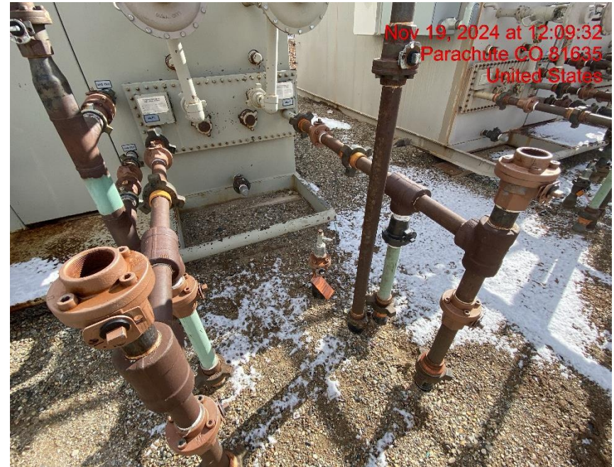
Open-Ended Lines on Separators – Photo #04976
