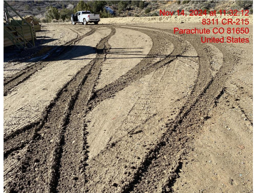
Lack of Stabilization – Photo #04930
