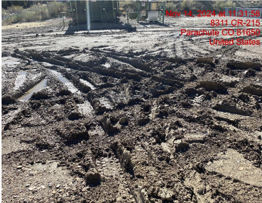
Lack of Stabilization – Photo #04929
