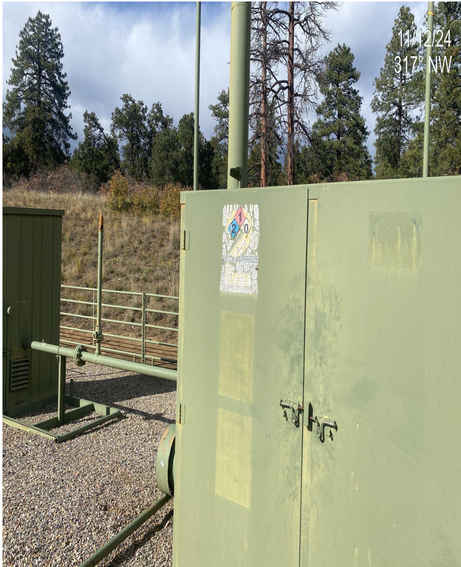
Photo 3. Placards at separator are deteriorating and illegible.
