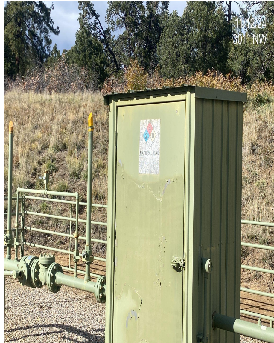
Photo 3. Placards at separator are deteriorating and illegible.
