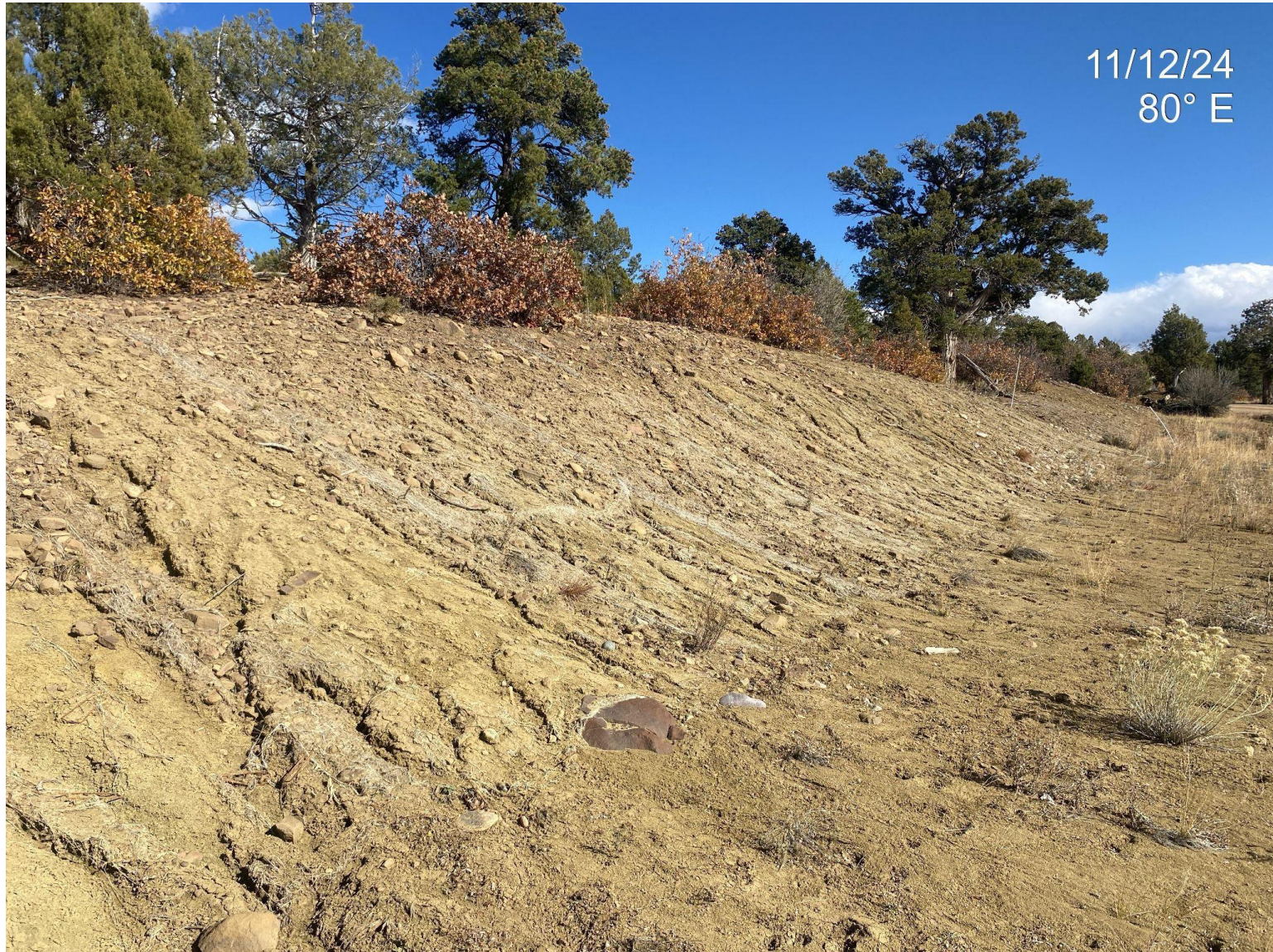
Photo 2. Location cut slope remains with bare soils and minimal vegetation and rill erosion. Erosion control blanket that was previously installed has since degraded.
