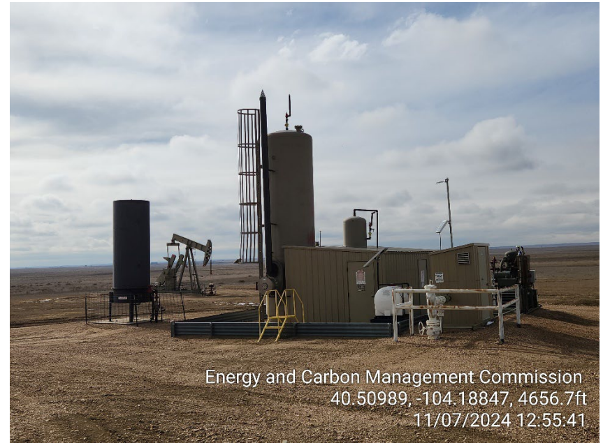
Photo 2 – Heater Treater and ECD
