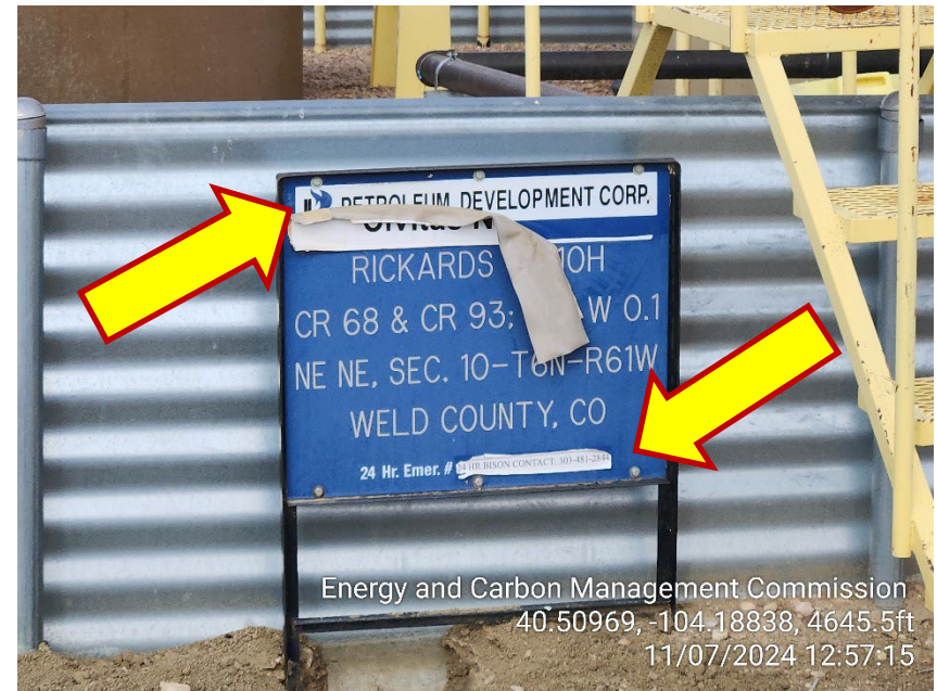
Photo 8 – Tank Battery Sign – Operator Name and 24 Hour Emergency Number NOT Current
