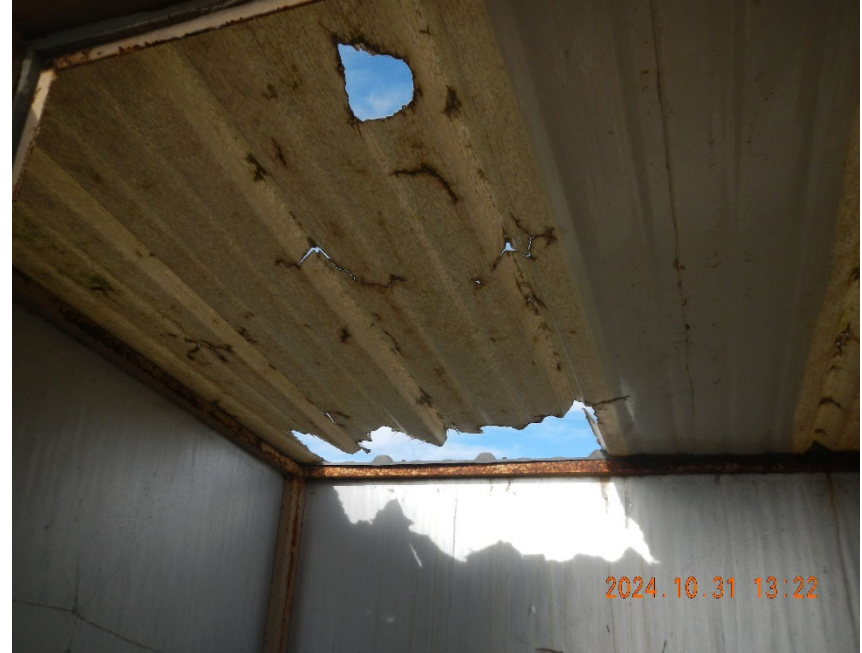
6. Hail damage to roof of meter shed.
