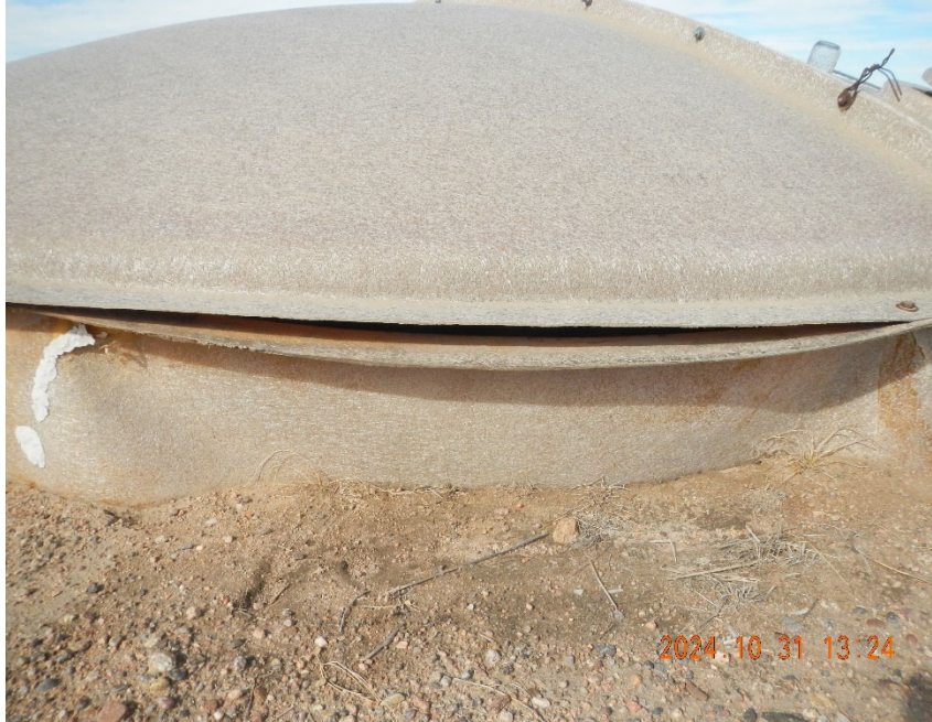
9. View of separation at the tank side wall and tank top.
