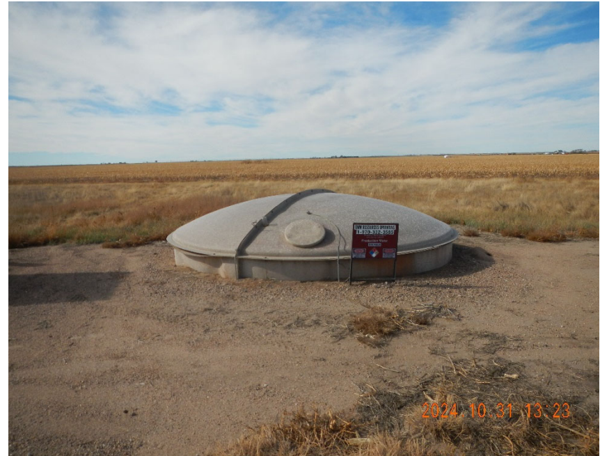
8. 200 bbl produced water tank at shared gathering location.
