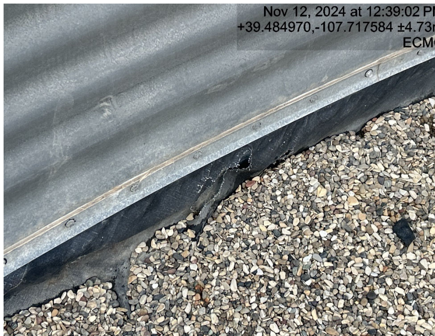
Holes in containment
