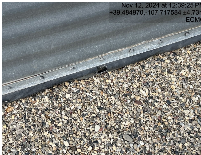
Holes in containment
