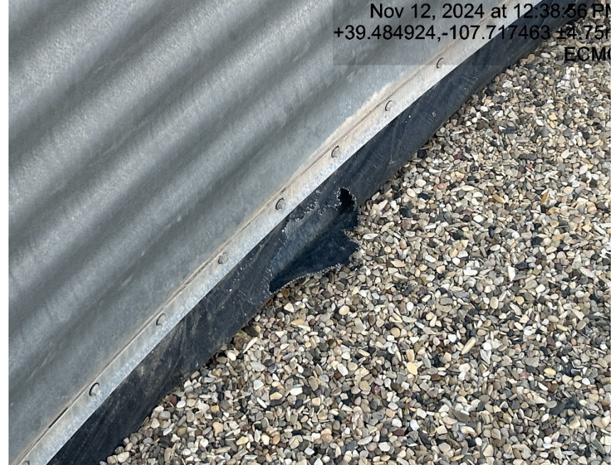
Holes in containment
