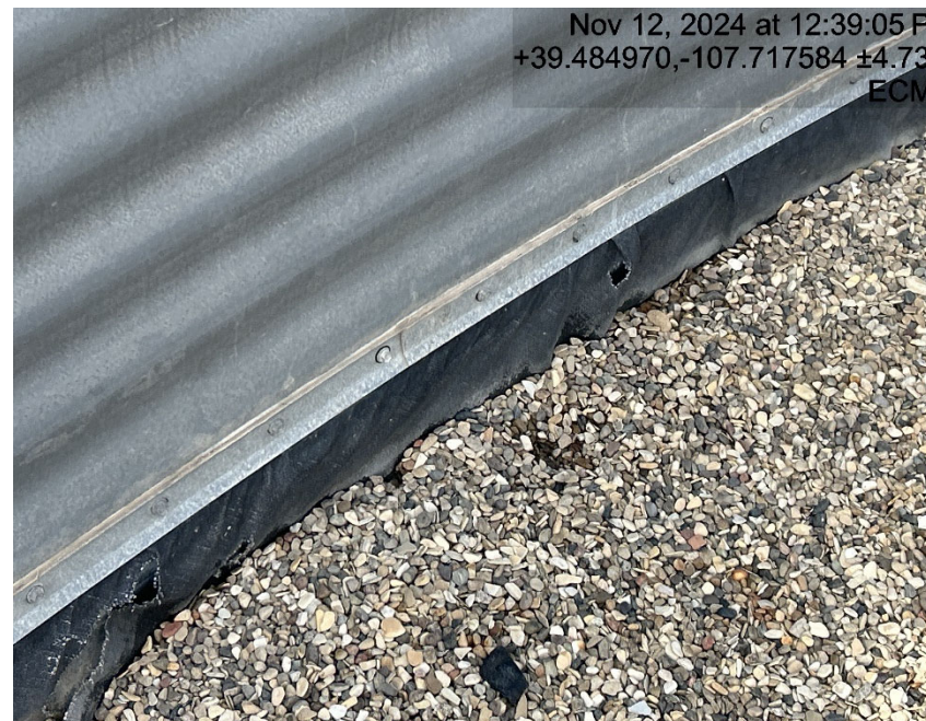
Holes in containment
