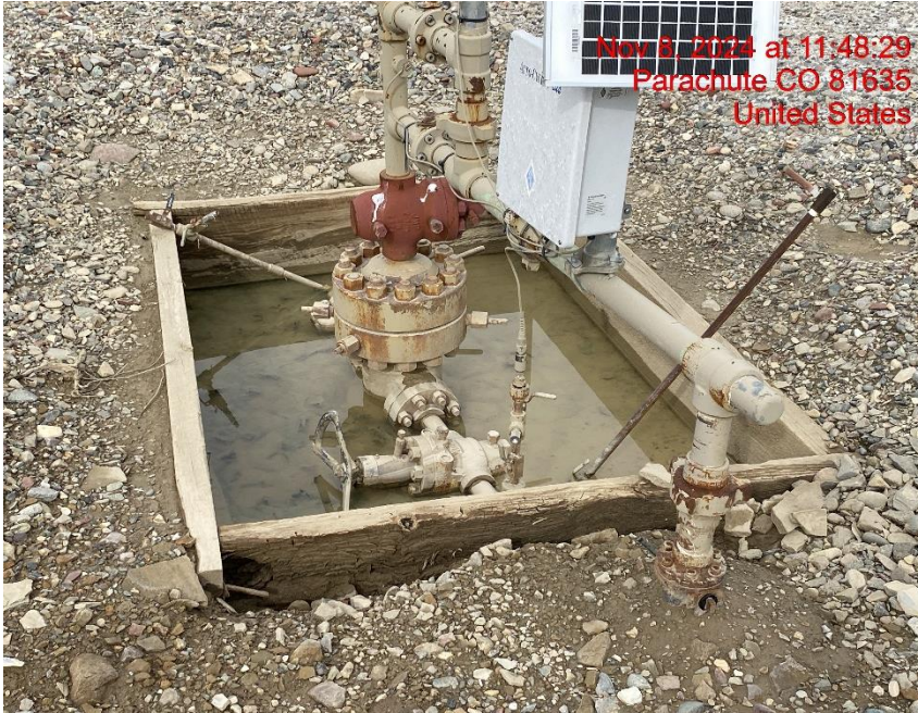
Open Wellhead Cellar/No Wildlife Egress – Photo #04803
