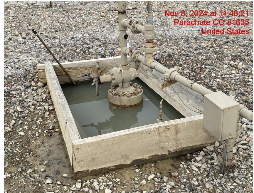
Open Wellhead Cellar/No Wildlife Egress – Photo #04802
