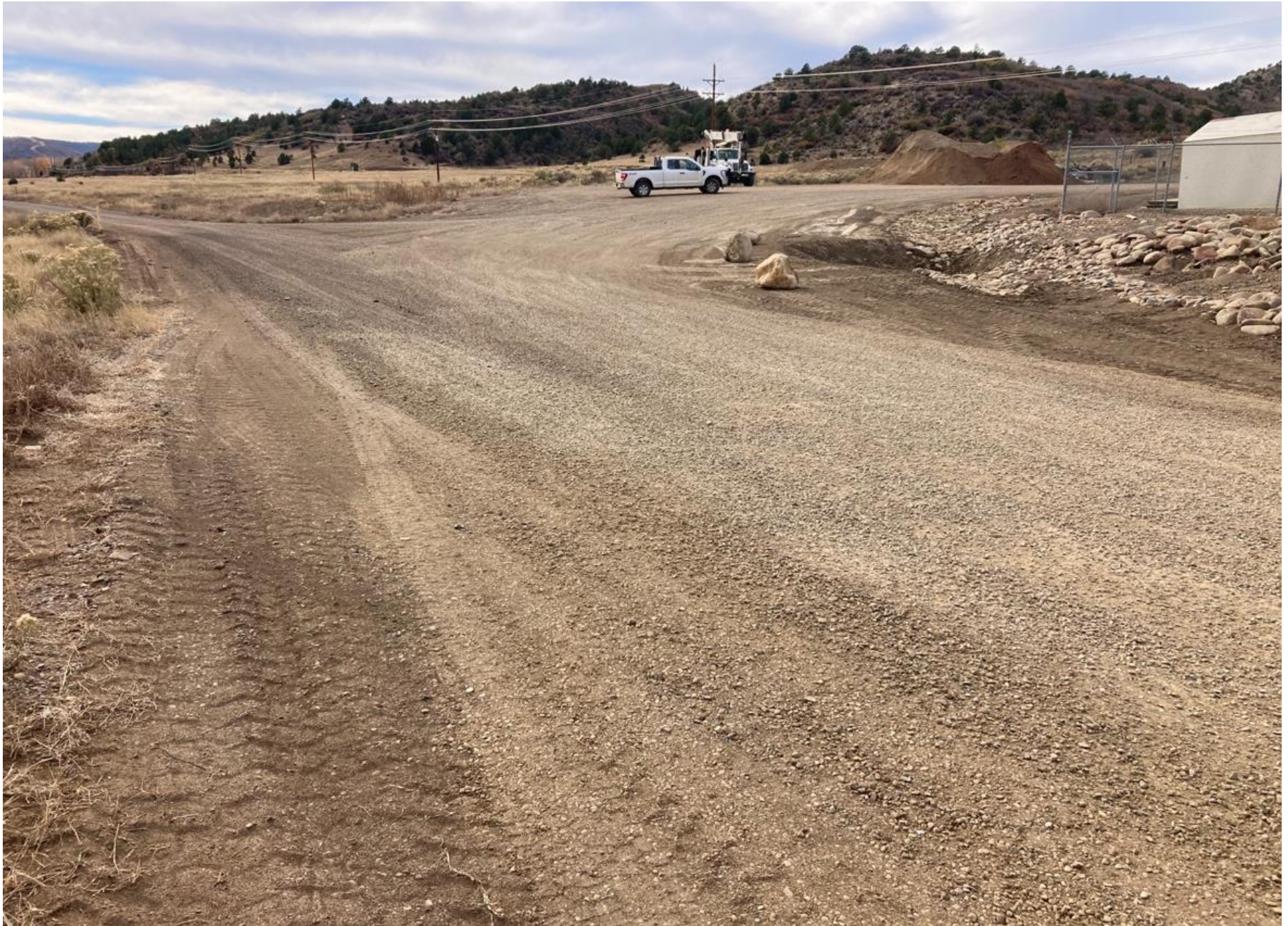
PHOTO 7: THE BLACK TOP PAVEMENT HAS BEEN REMOVED FROM THE MAIN ACCESS ROAD AND REPLACED WITH FRESH GRAVEL ROAD BASE. THE ACCESS ROAD HAS BEEN GRADED AND CROWNED TO PROMOTE STORMWATER SHEETFLOW TO THE DIVERSIONS.
