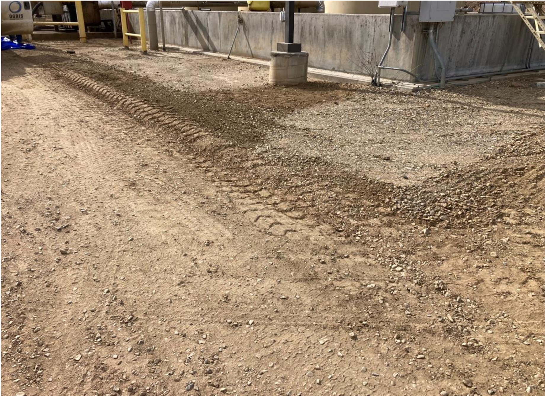
PHOTO 4: ALL STAINED SOIL ON LOCATION HAS BEEN REMOVED AND REPLACED WITH FRESH PAD MATERIAL.
