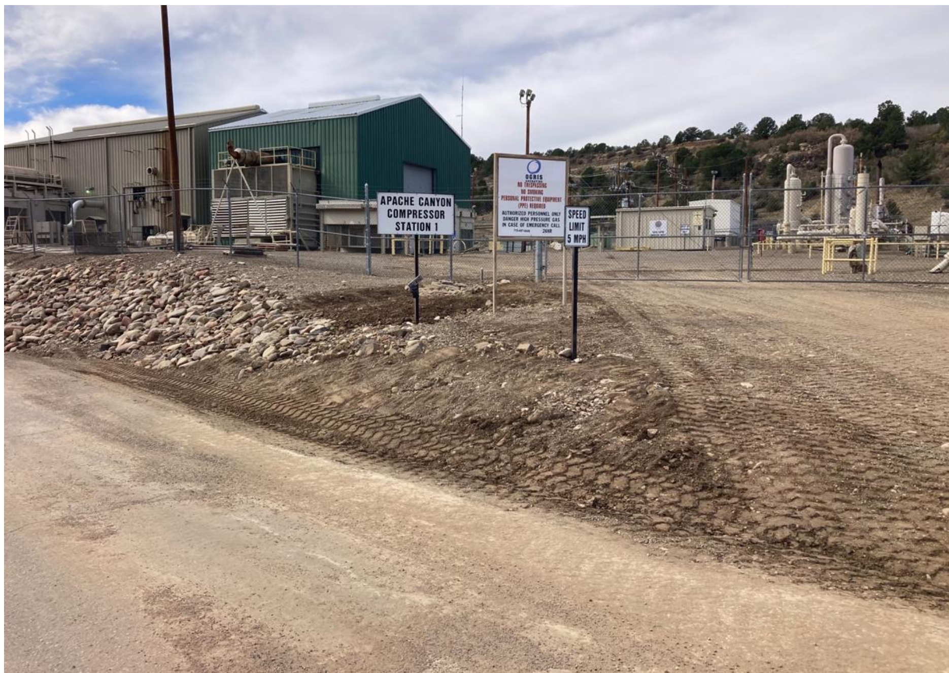
PHOTO 8: BMPs HAVE BEEN INSTALLED ON THE NORTH SIDE ACCESS. ALL DISTURBED AREAS HAVE BEEN TRACKED AND COMPACTED.
