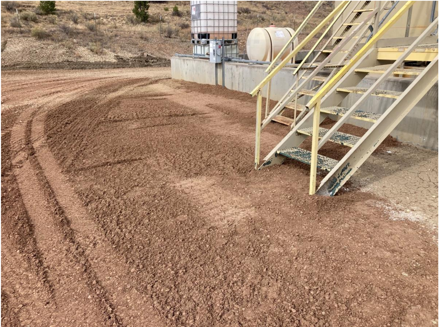
PHOTO 3: ALL STAINED SOIL ON LOCATION HAS BEEN REMOVED AND REPLACED WITH FRESH PAD MATERIAL.
