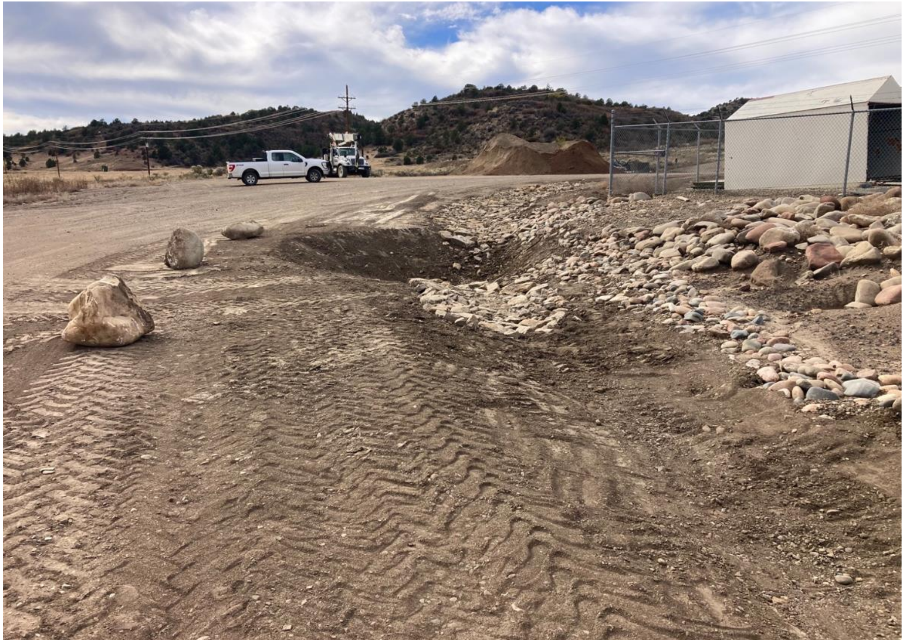
PHOTO 5: THE DIVERSION DITCH ALONG THE SOUTH SIDE ACCESS HAS BEEN REWORKED TO DIRECT STORMWATER ALONG THE ROAD AND INTO THE CULVERT BELOW. A LARGE SEDIMENT TRAP HAS BEEN CONSTRUCTED TO CONTAIN THE SILT MOVEMENT. THE ENTIRE AREA HAS BEEN TRACKED FOR COMPACTION.
