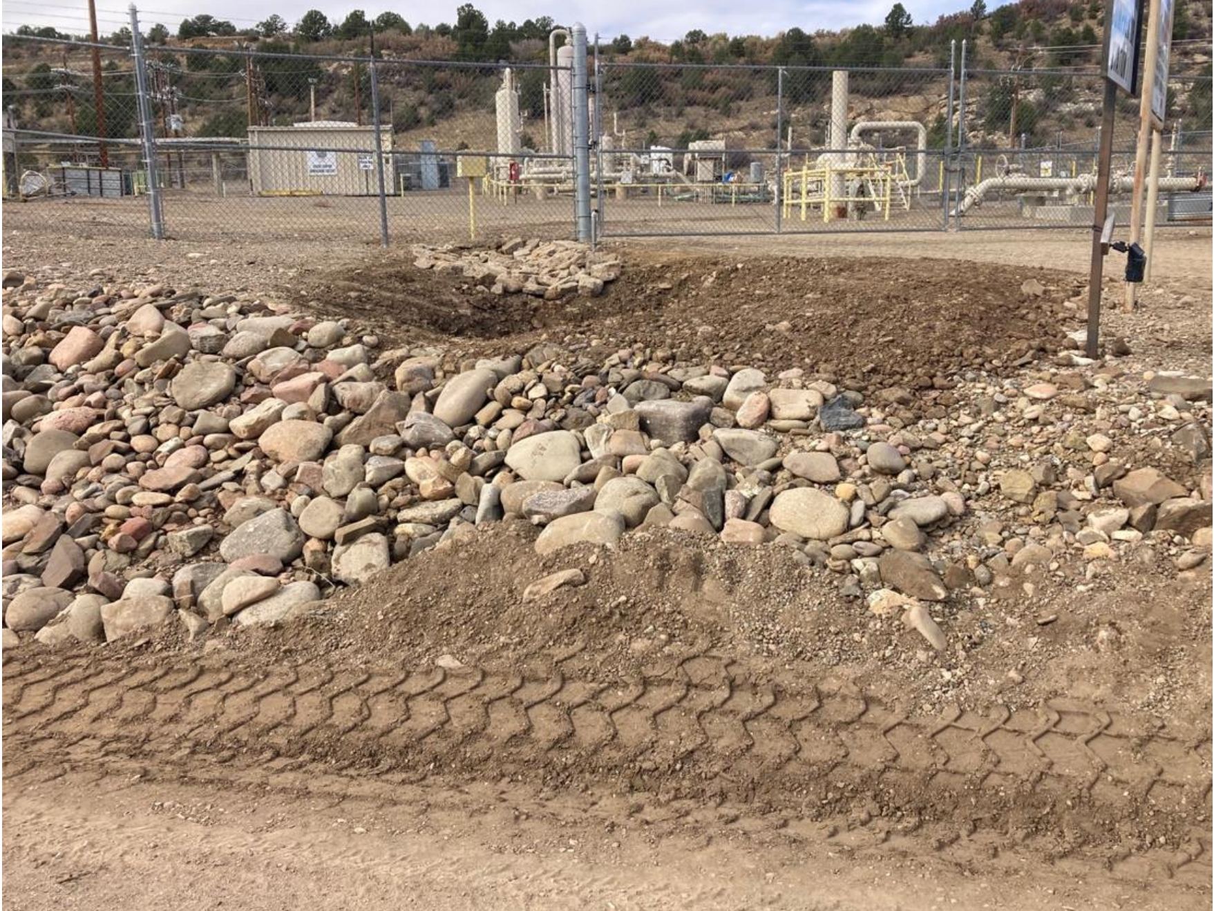
PHOTO 9: A ROCKED SPILLWAY AND SEDIMENT TRAP HAS BEEN INSTALLED.
