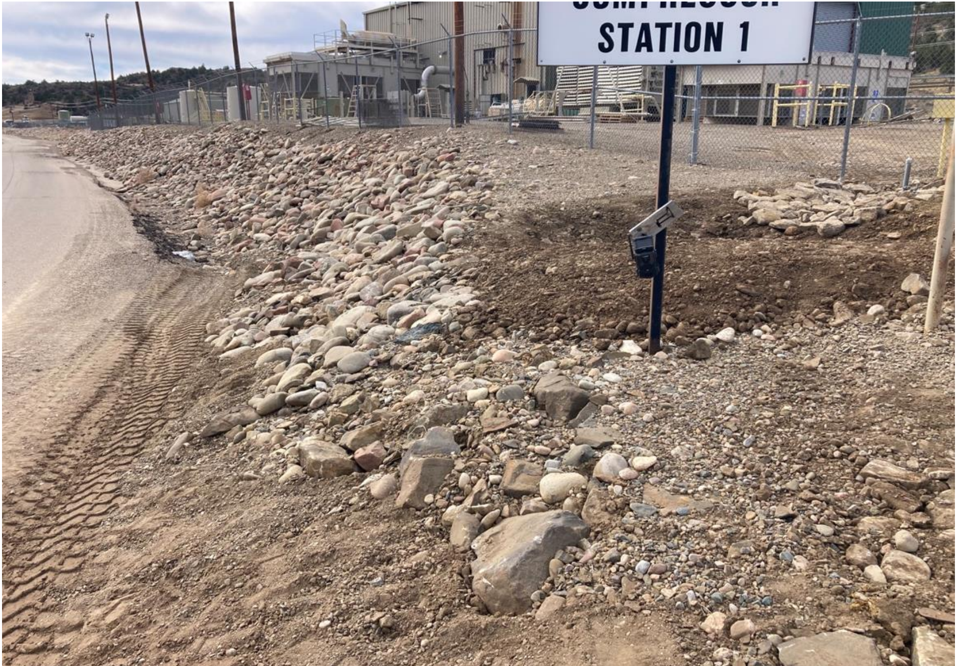
PHOTO 10: THE LOOSE SEDIMENT HAS BEEN CLEANED FROM THE ROADWAY AND THE DIVERSION DITCH REDEFINED TO SLOPE TO THE CULVERT.
