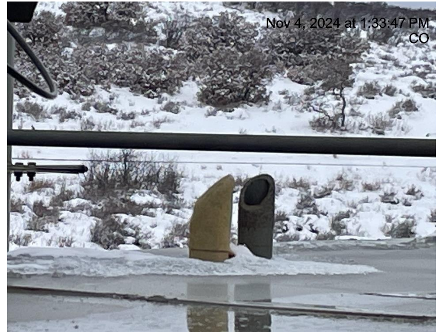
Photo # 8819 PRV vent line does not comply with CECMC pressure safety device rules
