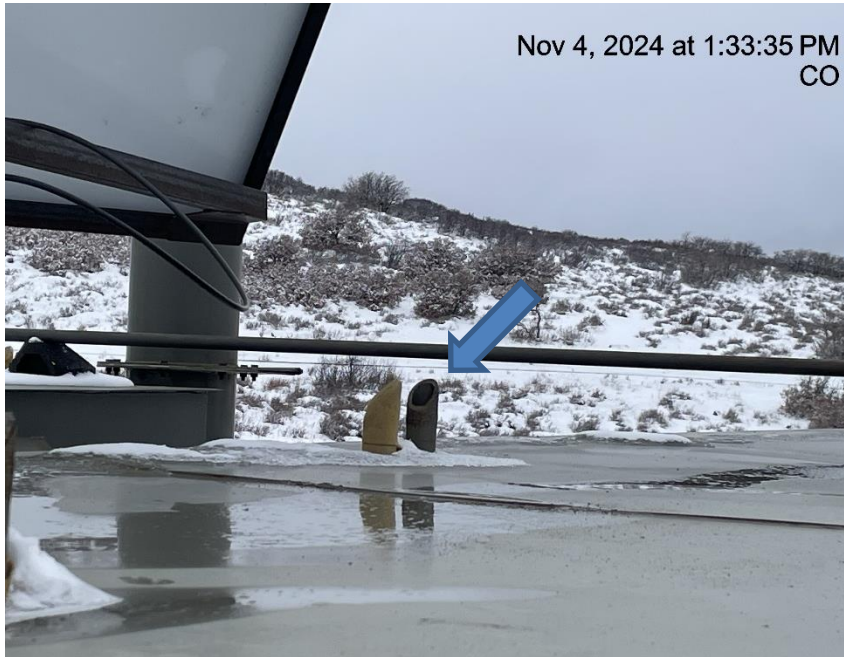
Photo # 8818 PRV vent line does not comply with CECMC pressure safety device rules
