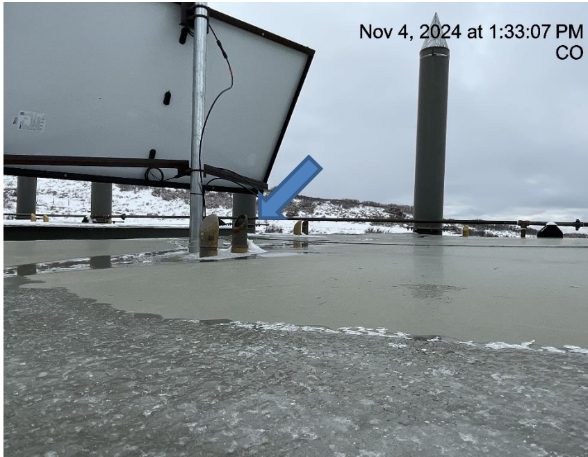
Photo # 8816 PRV vent line does not comply with CECMC pressure safety device rules
