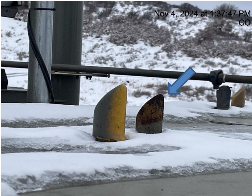
Photo # 8822 PRV vent line does not comply with CECMC pressure safety device rules
