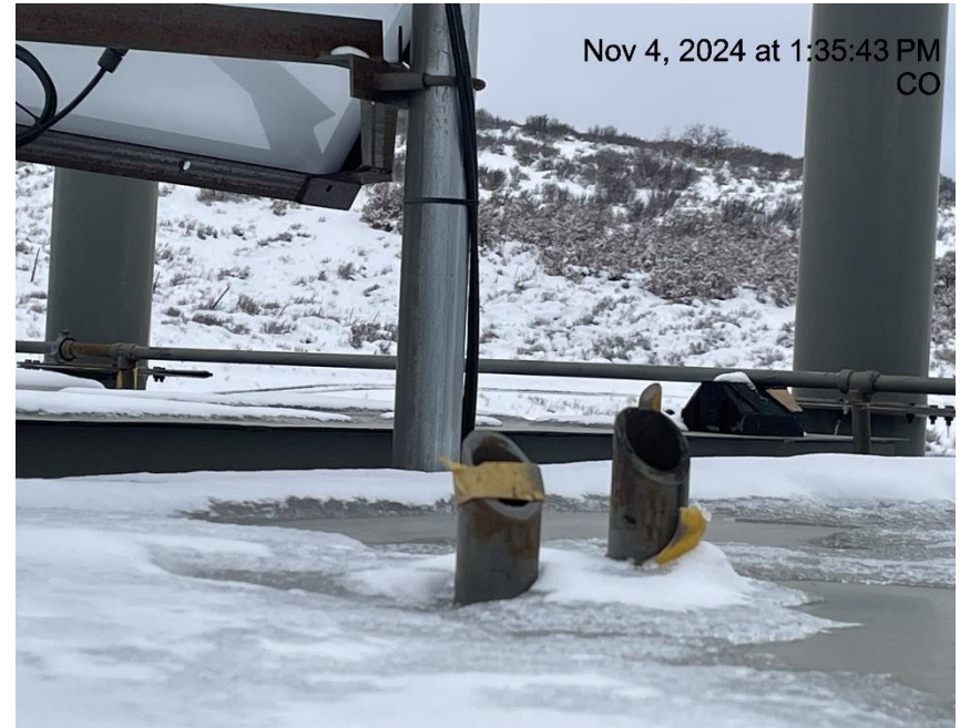
Photo # 8821 PRV vent line & rupture disc vent line do not comply with CECMC pressure safety device rules
