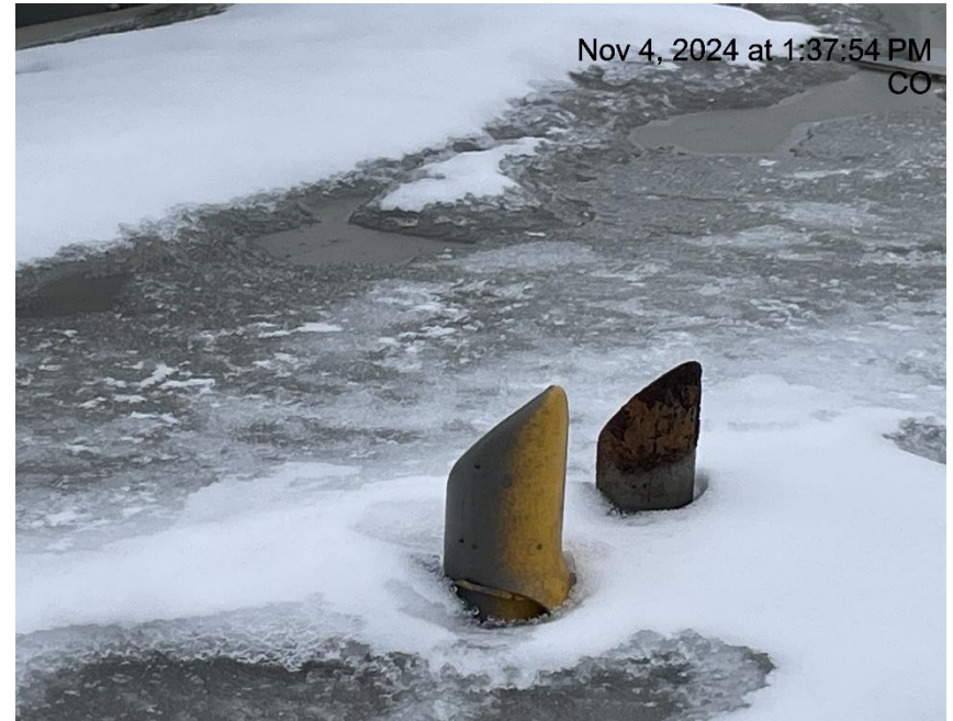
Photo # 8823 PRV vent line does not comply with CECMC pressure safety device rules
