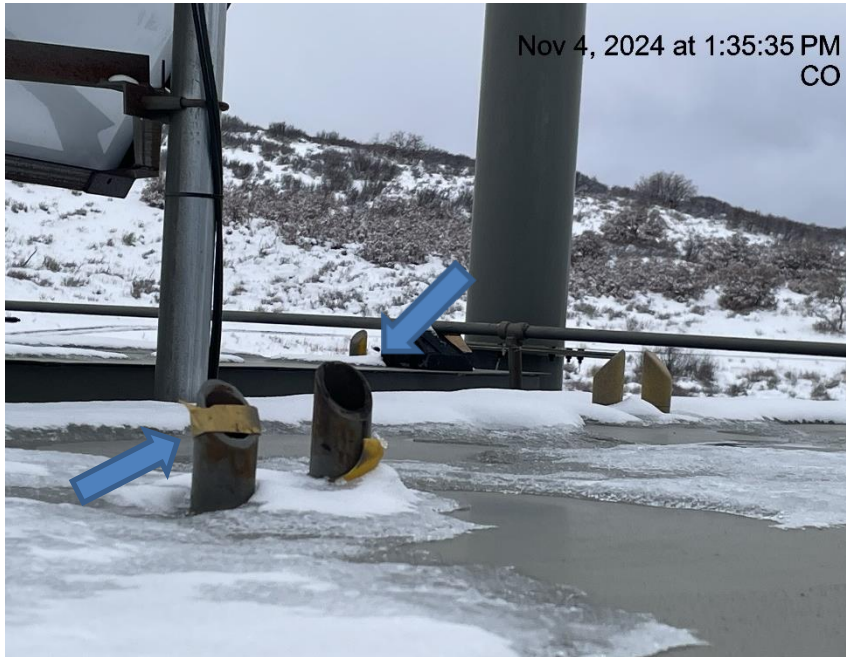
Photo # 8820 PRV vent line & rupture disc vent line do not comply with CECMC pressure safety device rules
