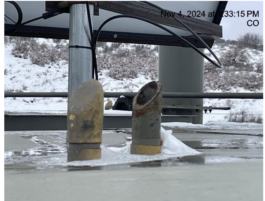
Photo # 8817 PRV vent line does not comply with CECMC pressure safety device rules
