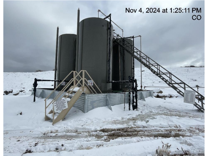
Photo # 8815 Tank battery contains three 500 bbl tanks – FORM 2A submitted by operator only lists 2 tanks/operator is not in compliance with CECMC rules
