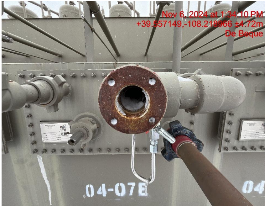
Photo # 8765 Open ended piping/wildlife hazard/ available for entry by wildlife
