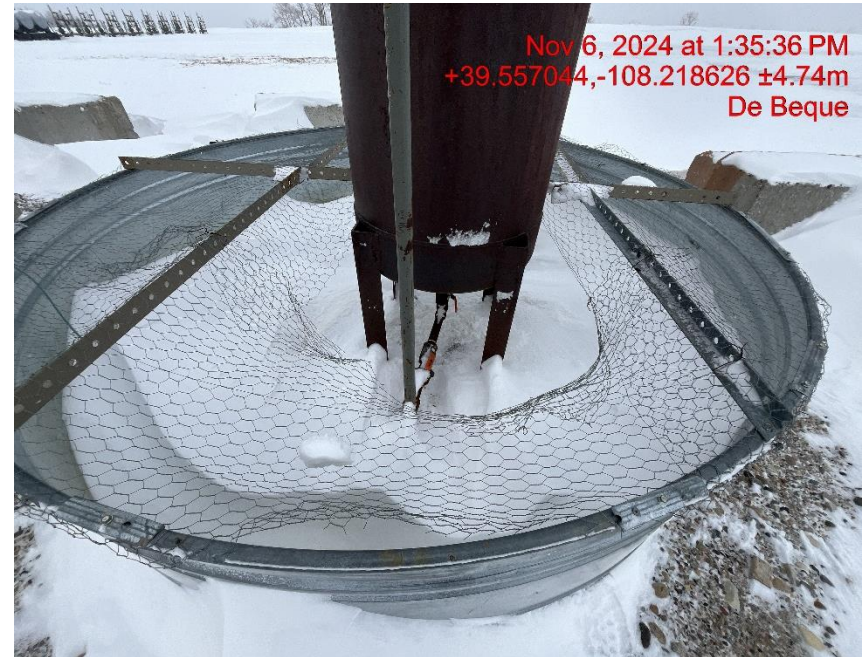
Photo # 8768 Wildlife protection for containment needs maintenance/screen is damaged
