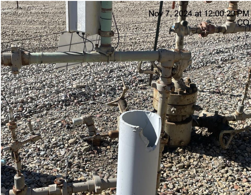
Photo # 9501 Open ended piping/wildlife hazard
