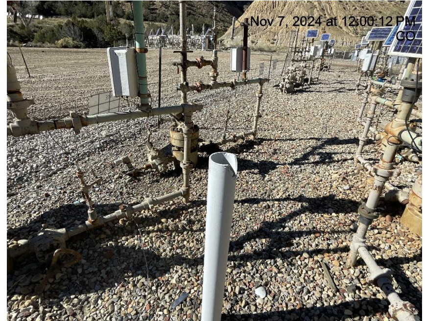
Photo # 9500 Open ended piping/wildlife hazard
