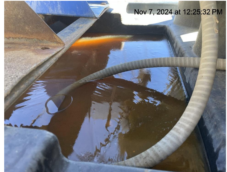
Photo # 9504 Failure to maintain chemical BMP - Chemical tank containment full of fluid/BMP insufficient to contain possible spill. (Additionally the standing fluid on top of chemical tank containment is also a wildlife hazard)
