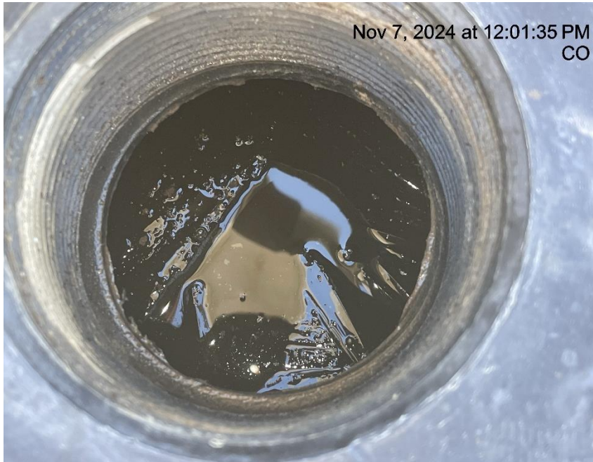
Photo # 9503 Failure to maintain chemical BMP - Chemical tank containment full of fluid/BMP insufficient to contain possible spill.
