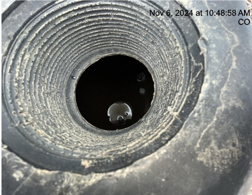
Photo # 9252 Failure to maintain chemical BMP – Chemical tank containment approximately 3/4 th full of fluid/BMP insufficient to contain possible spill
