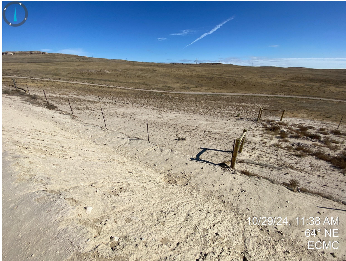
Photo 15. Erosion degradation on the eastern pit walls. Stormwater control measures/BMPs remain inadequate at this location.
