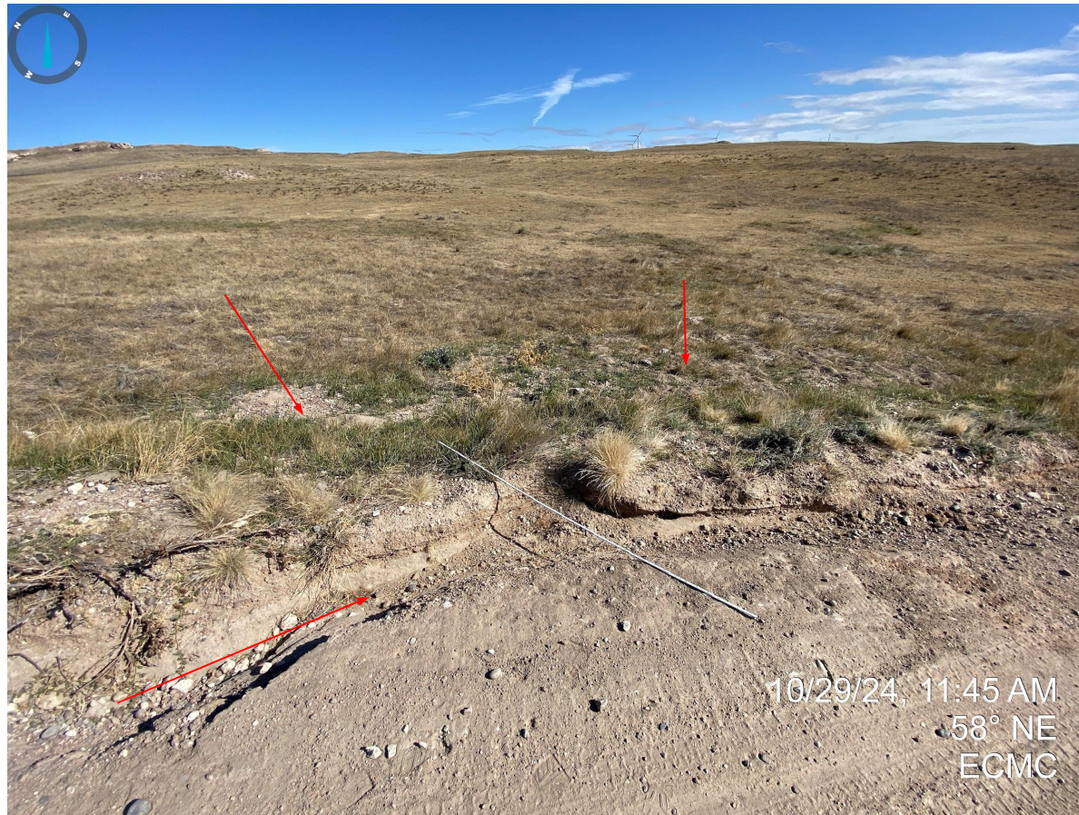
Photo 4. Sediment deposition and erosion degradation along the access road, east of pit.
