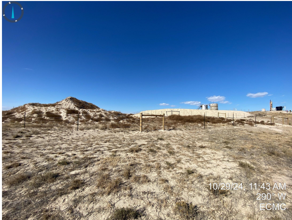
Photo 9. Taken southeast of the excavated area and stockpiled material; no apparent perimeter stormwater control measures and sediment deposition observed.
