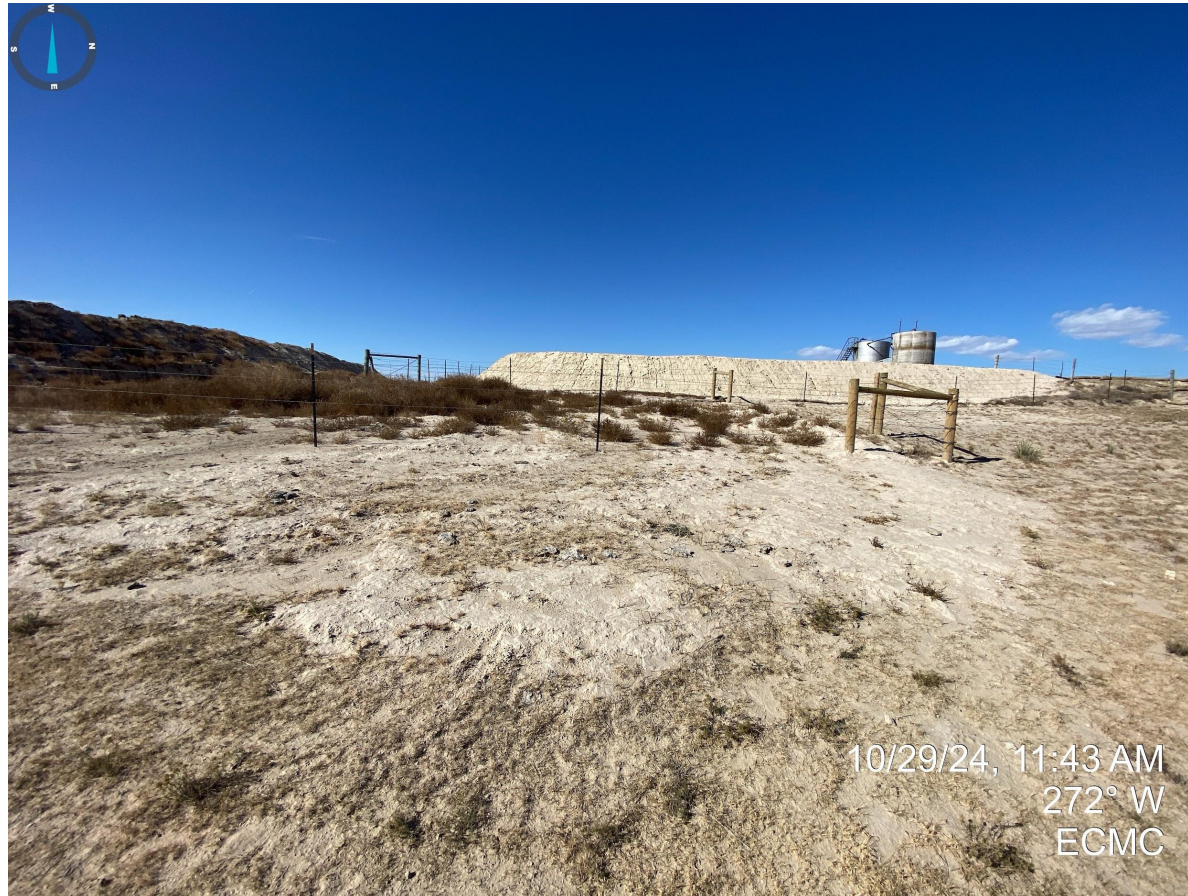
Photo 10. Sediment deposition resulting from unstabilized soils, southeast corner of the pit.
