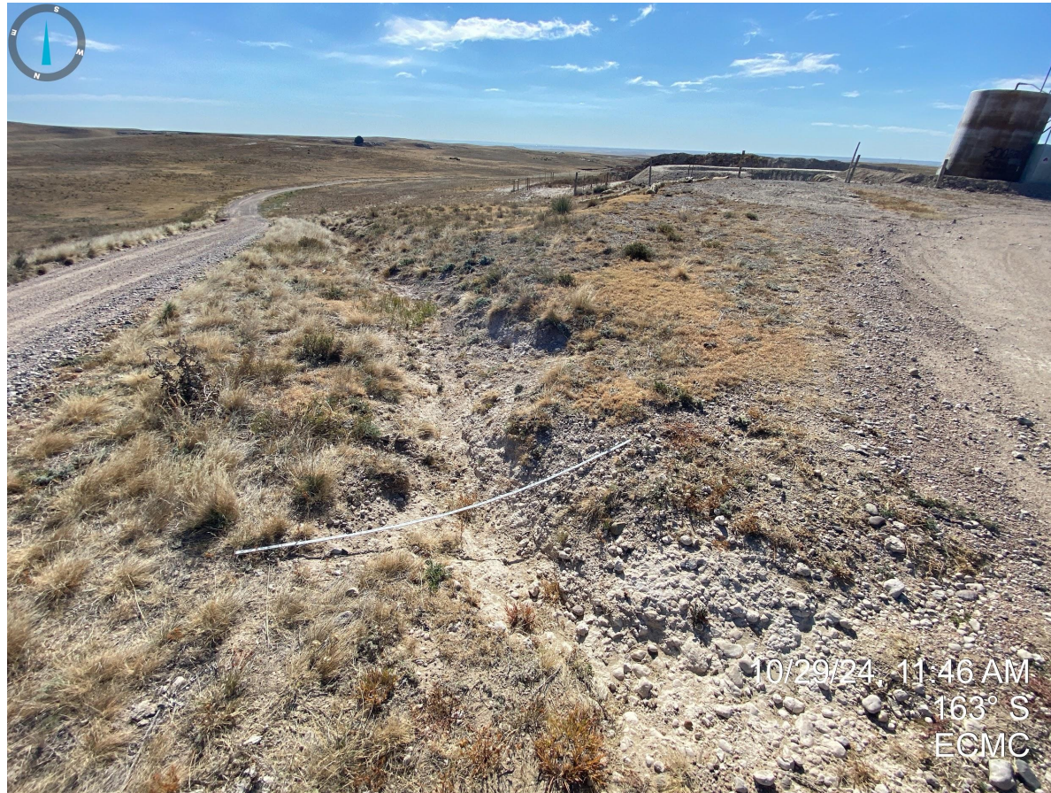
Photo 1. Taken north of pit. Evidence of erosion degradation, previously documented, does not appear to have been repaired/stabilized with no evidence of control measures/BMPs observed that would prevent further erosion of the production areas and access roads.
