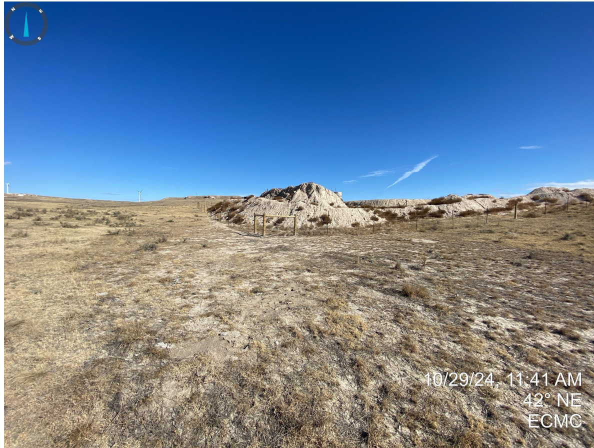
Photo 7. Sediment deposition resulting from unstabilized stockpiles, southwest corner of the pit.
