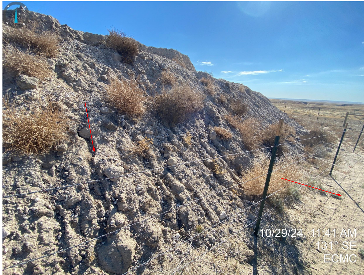
Photo 6. Continued from Photo 5; evidence of unstabilized soils (rill erosion) and sediment migration outside of the fenced portions. Undesirable vegetation (russian thistle) also observed.
