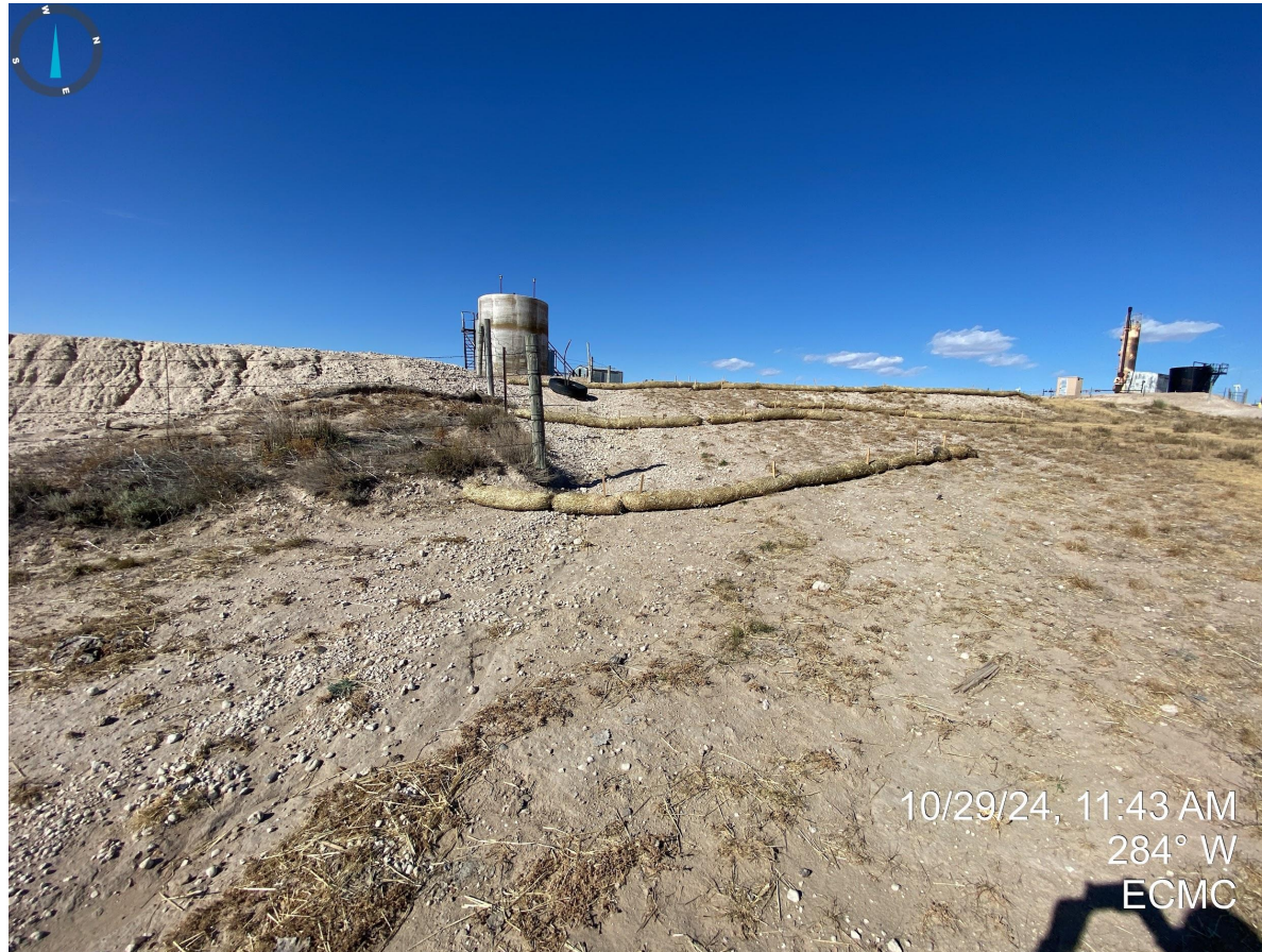
Photo 12. Erosion degradation occurring on the northern/eastern portion of the production areas, near the pit. Stormwater control measures appear to have been reinstalled, however, they don't not appear to be installed per good engineering practices (e.g. trenched and backfilled).
