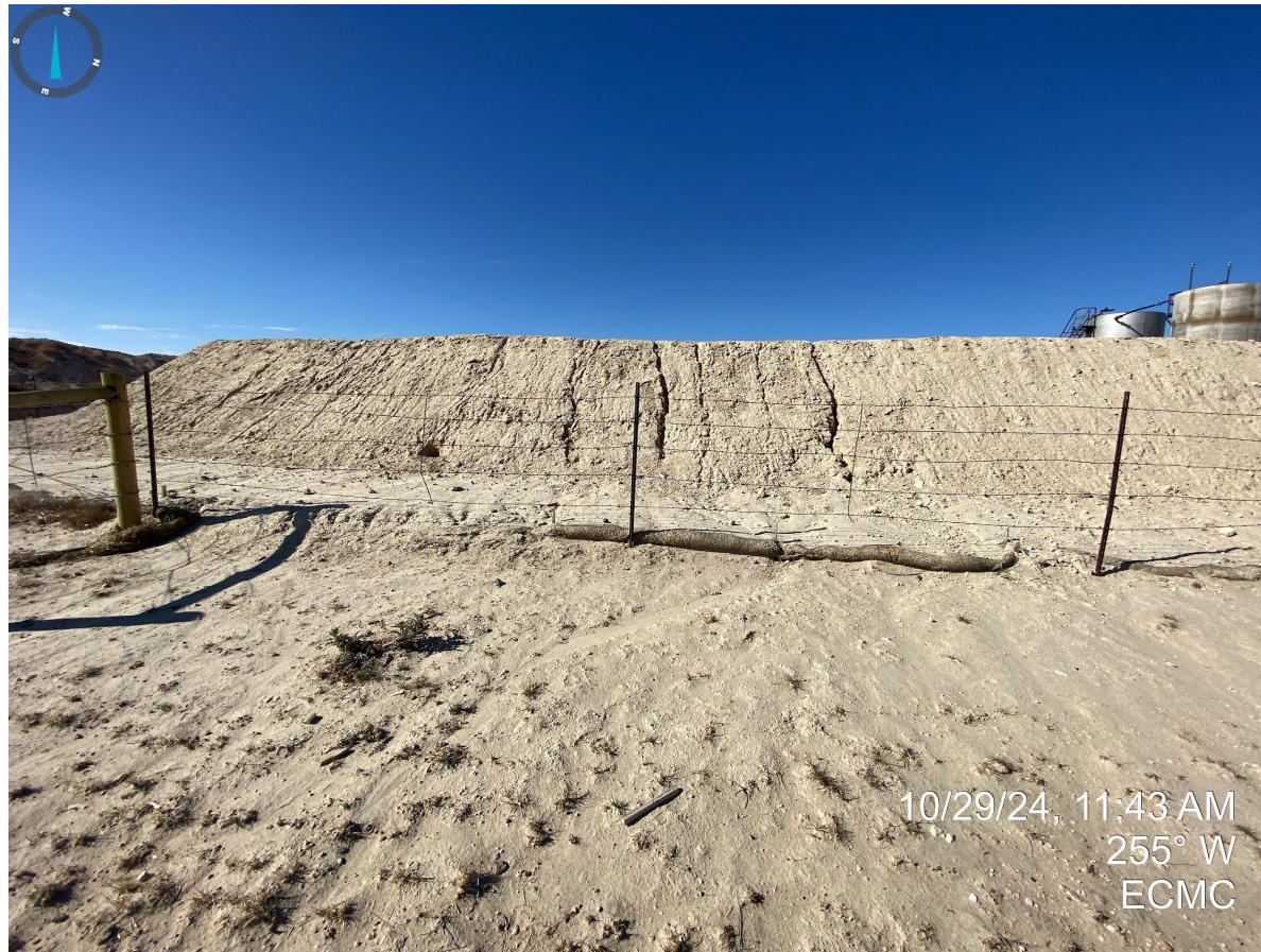
Photo 11. Sediment deposition resulting from unstabilized soils, eastern portion of the pit. Stormwater control measures remain inadequate at this location.
