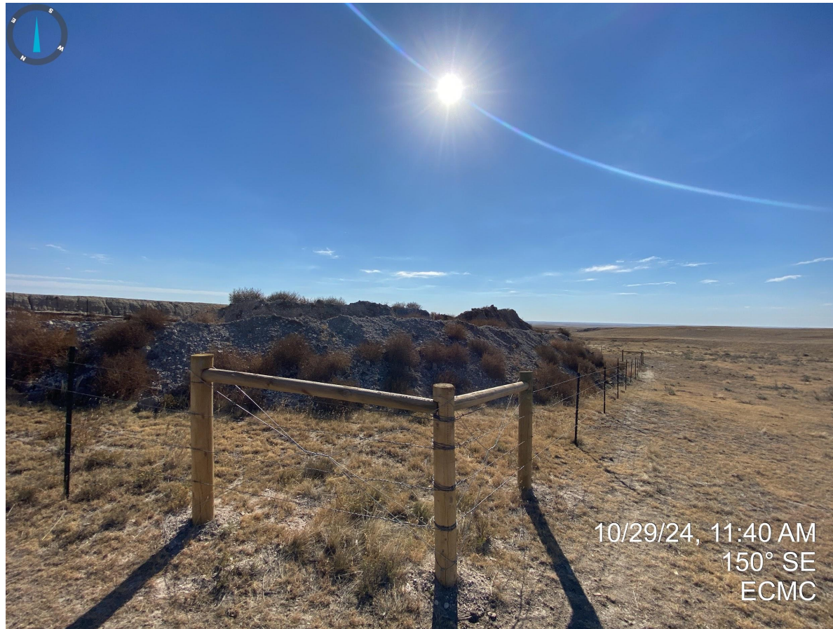
Photo 5. Taken from the north side of the stockpiled soils. No perimeter stormwater control measures/BMPs, or impermeable liners underneath the stockpile were observed during this inspection. Impacted soils appear to have been placed directly on top of undisturbed lands. Additionally, it does not appear that topsoil has been salvaged Per Rule 1002.b prior to stockpiling the soil on undisturbed portions of land. Undesirable vegetation observed throughout stockpiled areas.
