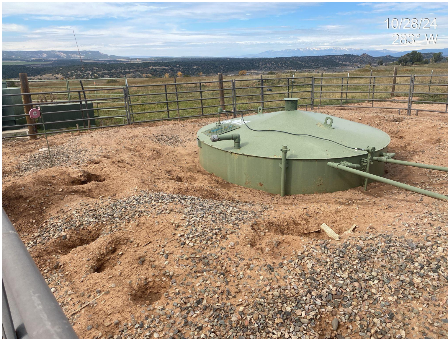
Photo 4. Produced water tank secondary containment/berm has been compromised by Burrows and erosion and is not longer functioning to its full capacity.
