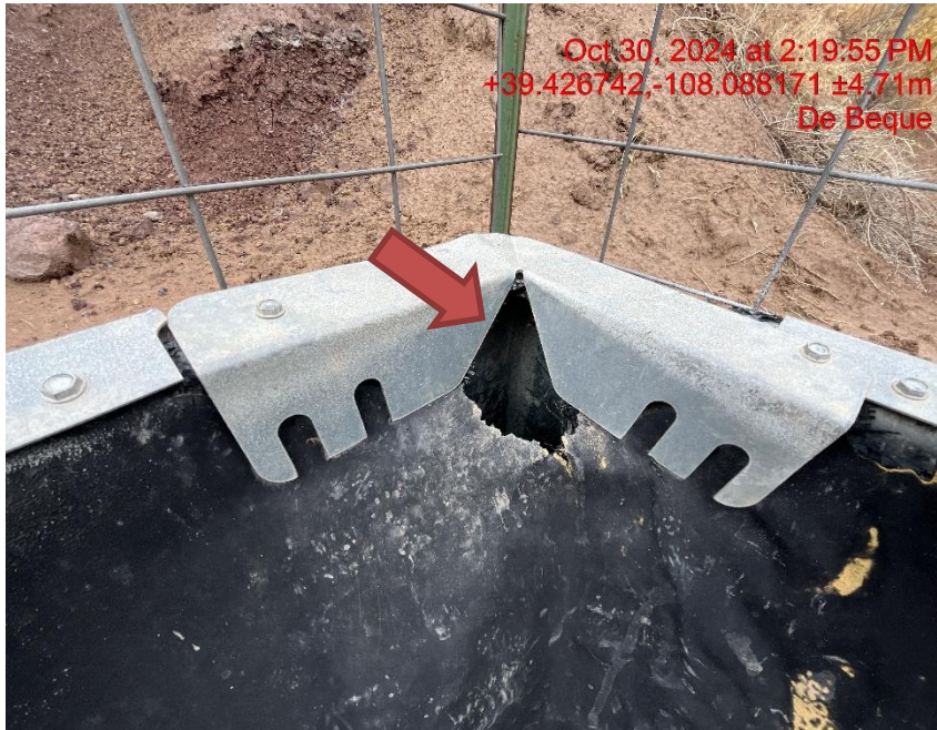
Photo # 8424 Hole in secondary containment/liner needs maintenance
