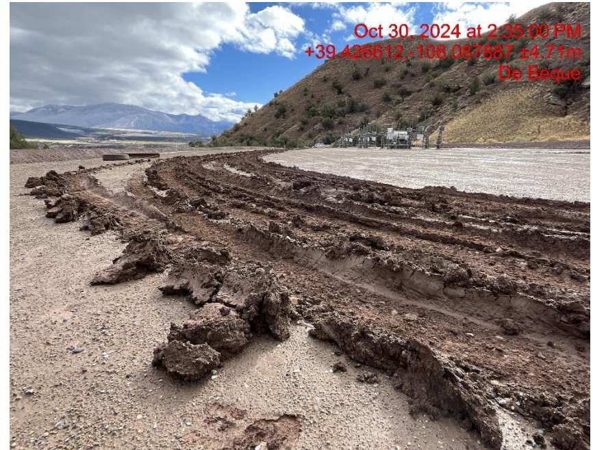
Photo # 8441 Lack of stabilization/compaction on location/insufficient tracking BMP's
