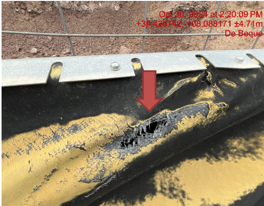
Photo # 8426 Hole in secondary containment/liner needs maintenance
