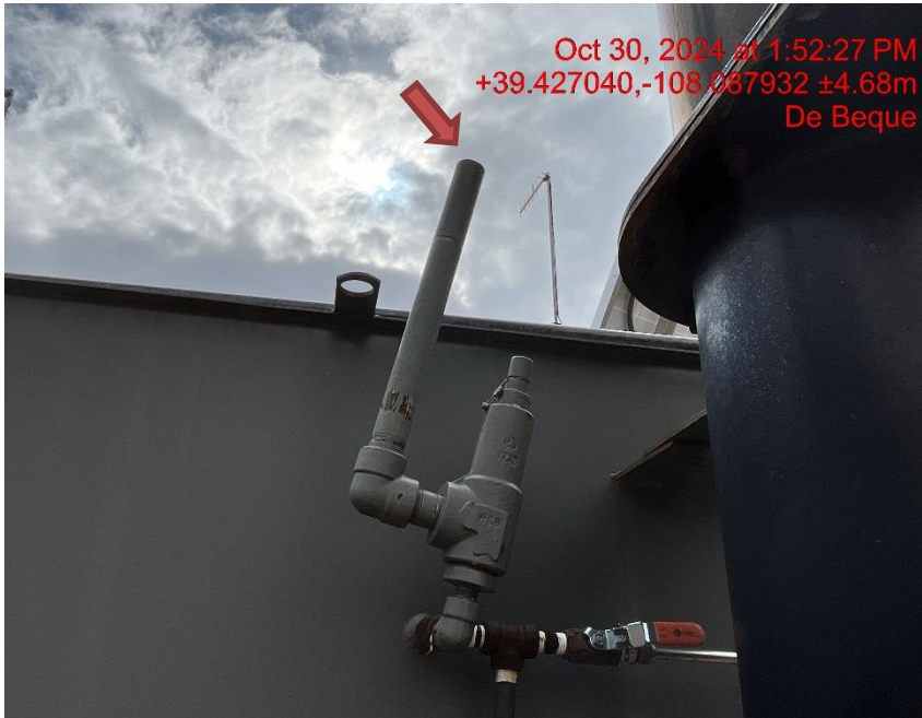
Photo # 8394 PRV vent line does not comply with CECMC pressure safety device rules
