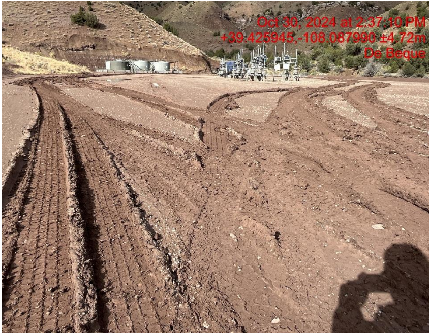
Photo # 8443 Lack of stabilization/compaction on location/insufficient tracking BMP's
