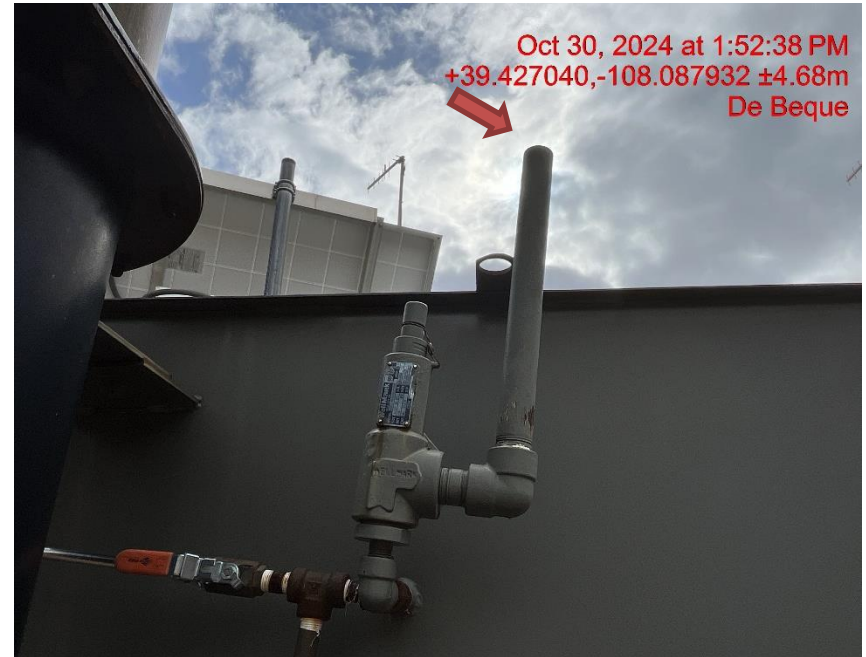
Photo # 8395 PRV vent line does not comply with CECMC pressure safety device rules
