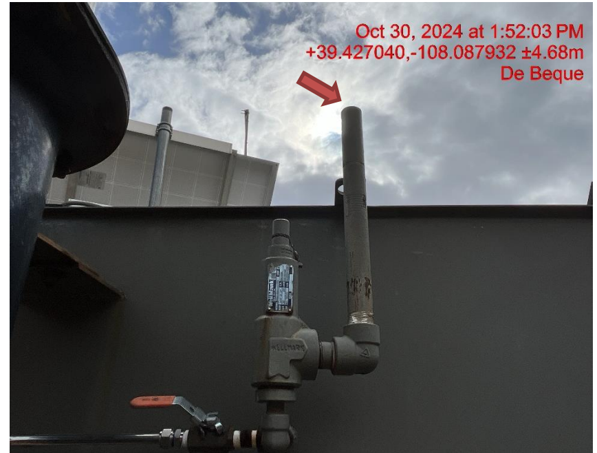
Photo # 8393 PRV vent line does not comply with CECMC pressure safety device rules
