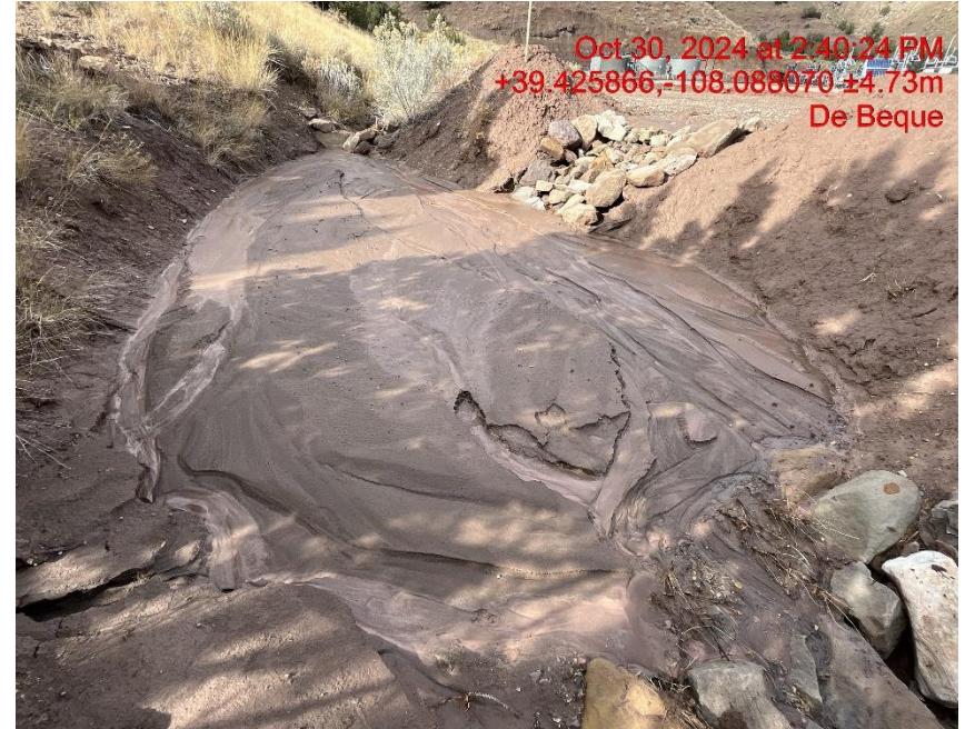
Photo # 8449 Sediment trap needs maintenance
