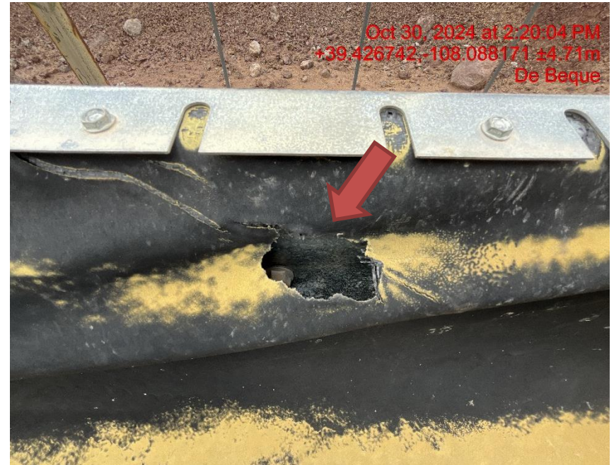
Photo # 8425 Hole in secondary containment/liner needs maintenance
