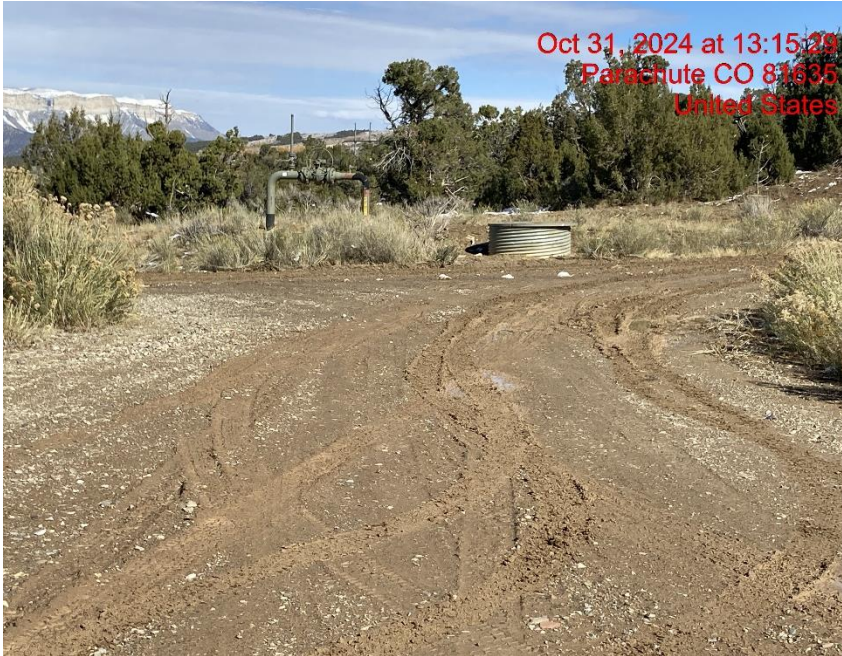
Insufficient Tracking BMPs – Photo #04664
