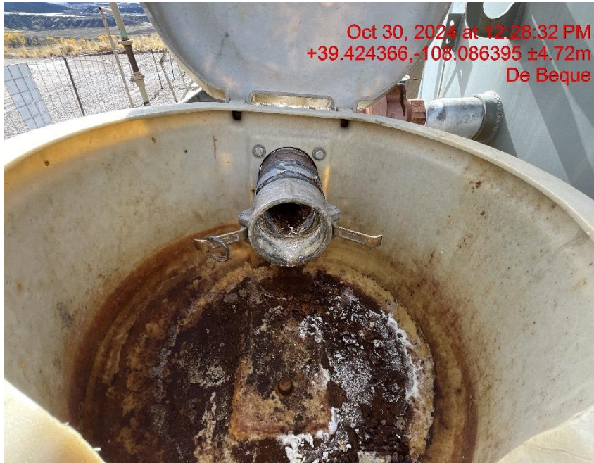
Photo # 8353 Open ended load line
