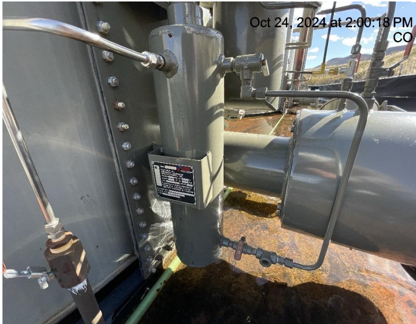
Photo # 7264 PRV vent line on tank heater does not comply with CECMC pressure safety device rules
