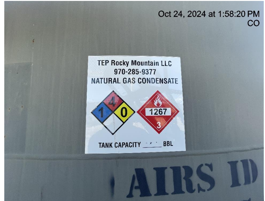
Photo # 7265 Tank capacity on label illegible/does not comply with CECMC tank labeling rules
