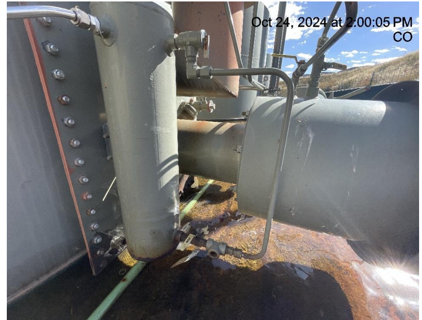
Photo # 7263 PRV vent line on tank heater does not comply with CECMC pressure safety device rules
