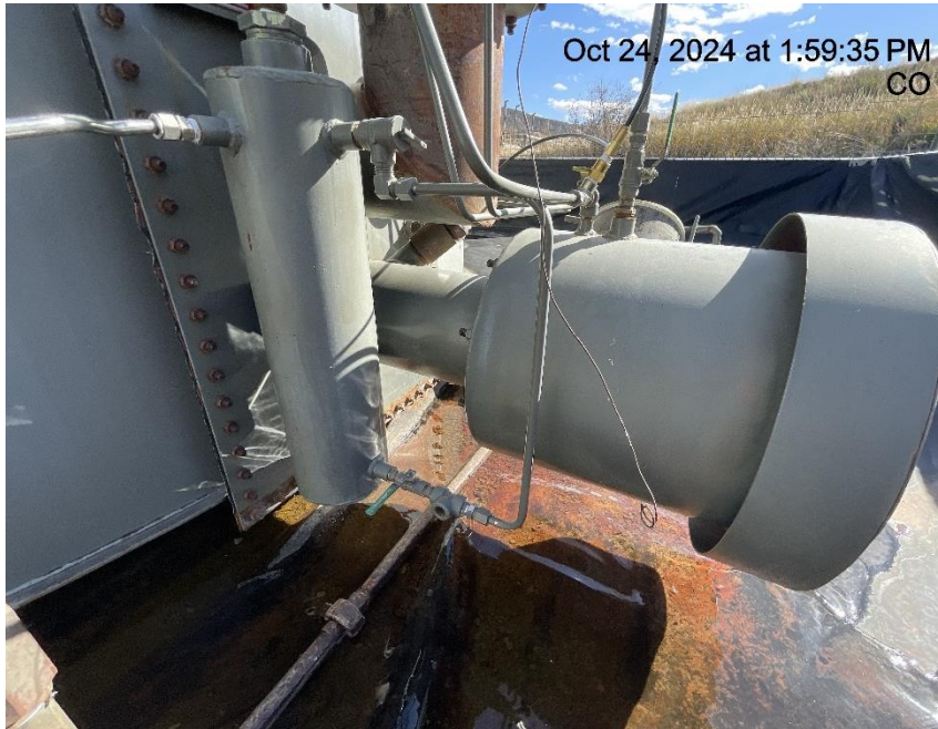
Photo # 7262 PRV vent line on tank heater does not comply with CECMC pressure safety device rules
