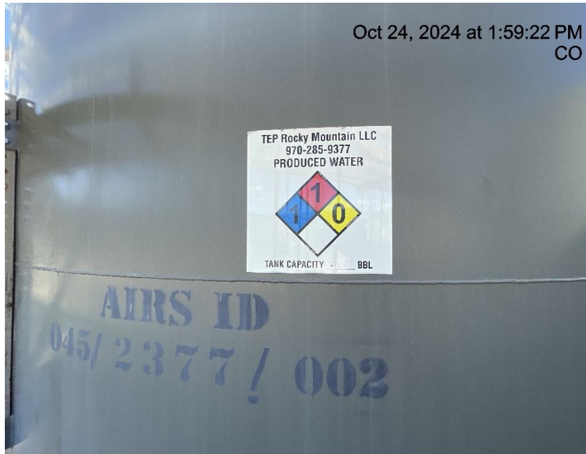
Photo # 7268 Tank capacity on label illegible/does not comply with CECMC tank labeling rules
