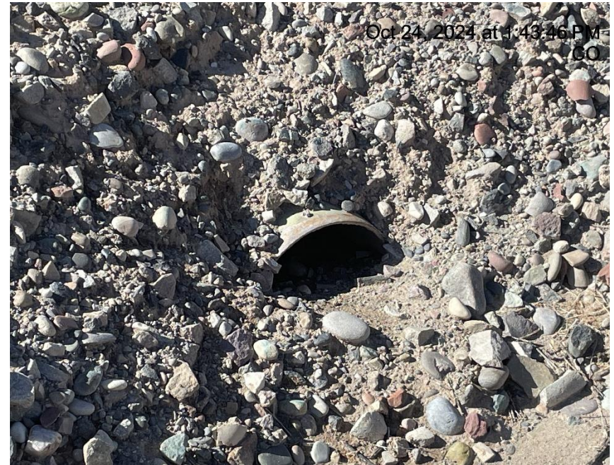
Photo # 7271 Large amount of sediment buildup at culvert outlet/capacity reduced/may need maintenance in near future
