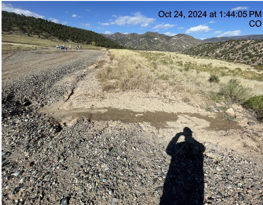
Photo # 7270 Large amount of sediment buildup at culvert outlet/capacity reduced/may need maintenance in near future
