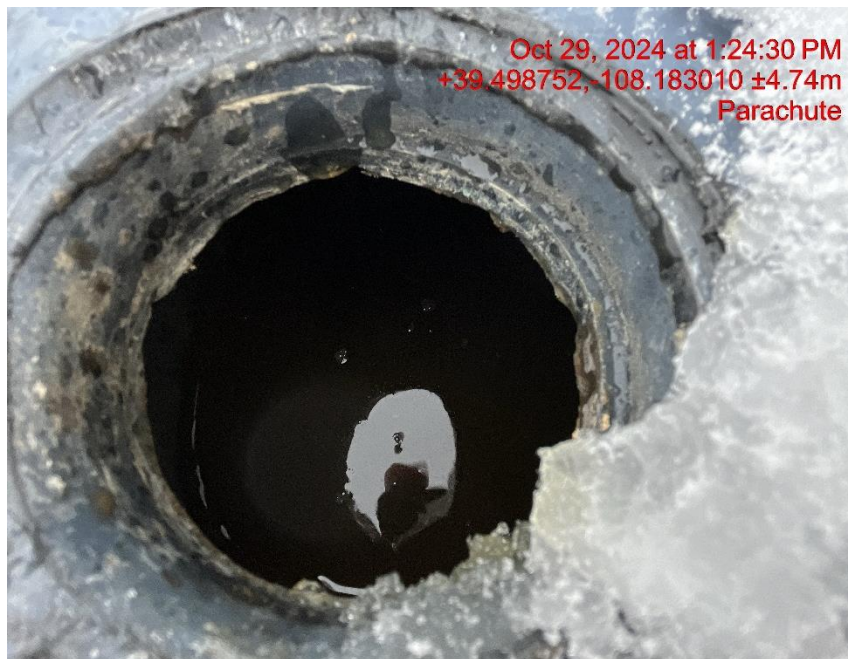
Photo # 8227 Failure to maintain chemical BMP's/chemical containments full of fluid & not sufficient to contain possible spill
