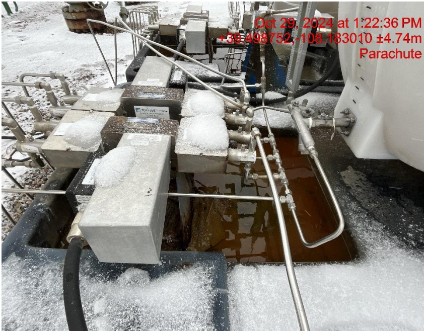
Photo # 8220 Failure to maintain chemical BMP's/chemical containments full of fluid & not sufficient to contain possible spill
