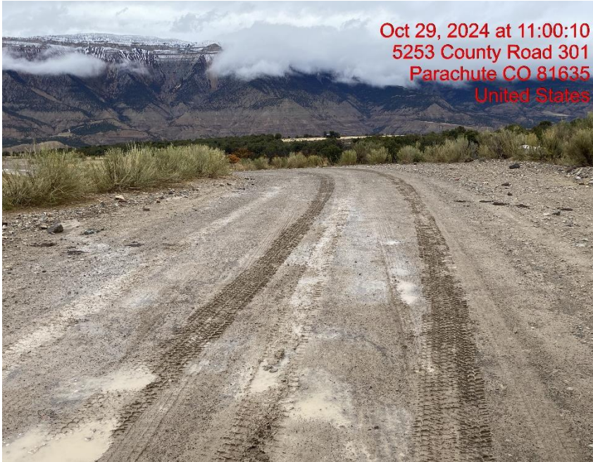
Insufficient Tracking BMPs – Photo #04547
