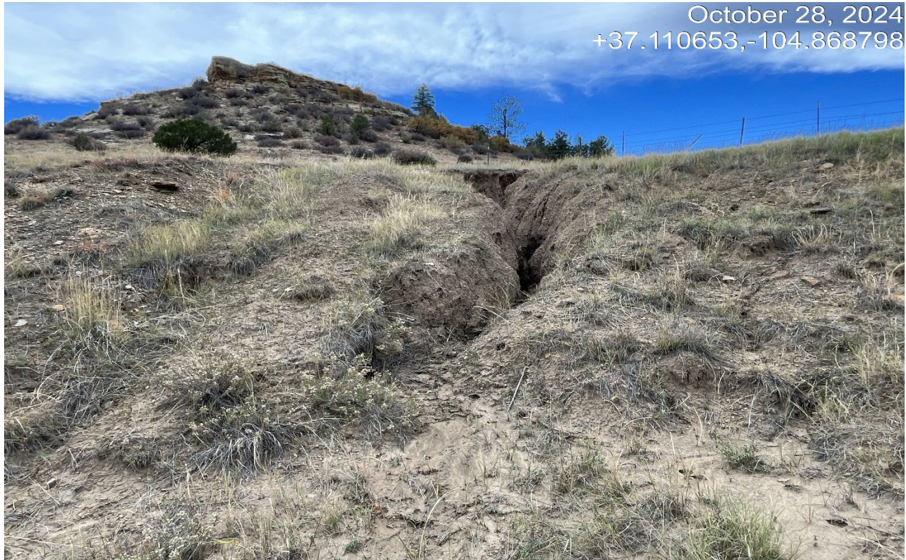
Photo 3. Facing west toward the cut slope. This erosion gully needs to be repaired and stabilized.
