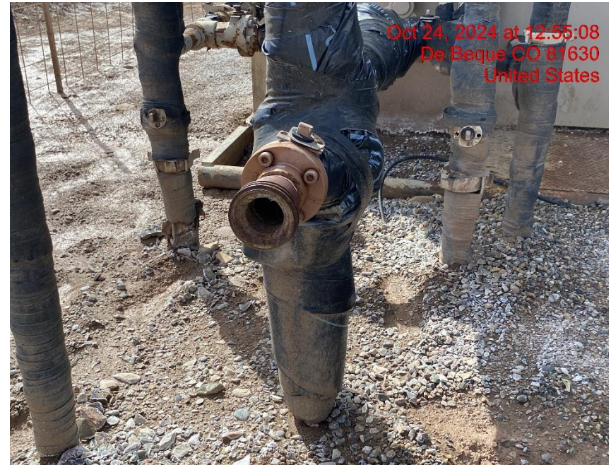
Open-Ended Line on Separators – Photo #04523
