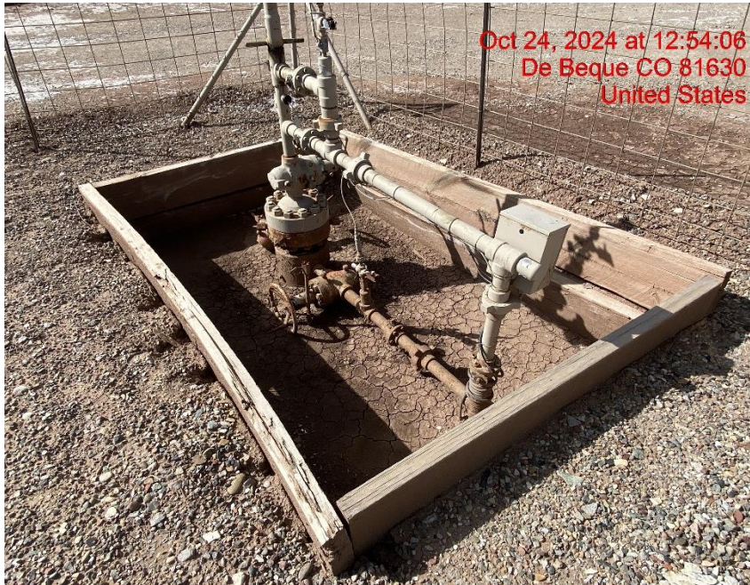
Open Wellhead Cellar/No Wildlife Egress – Photo #04519
