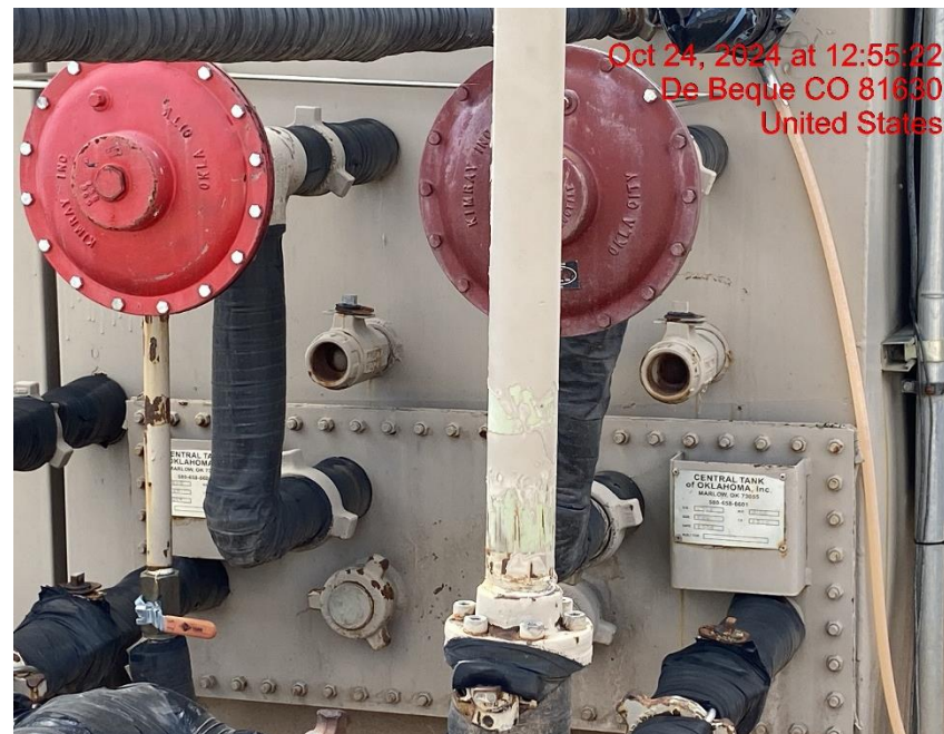
Open-Ended Lines on Separators – Photo #04525
