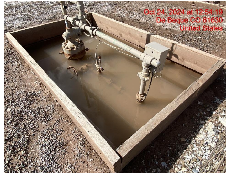
Open Wellhead Cellar/No Wildlife Egress – Photo #04520
