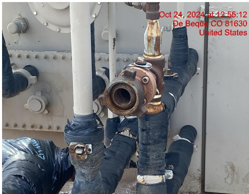
Open-Ended Line on Separators – Photo #04524
