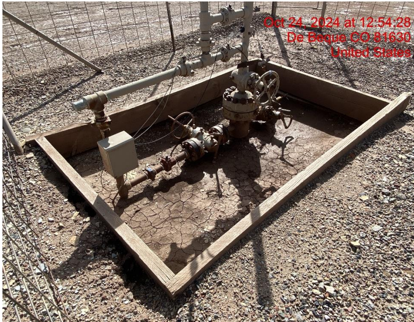
Open Wellhead Cellar/No Wildlife Egress – Photo #04521
