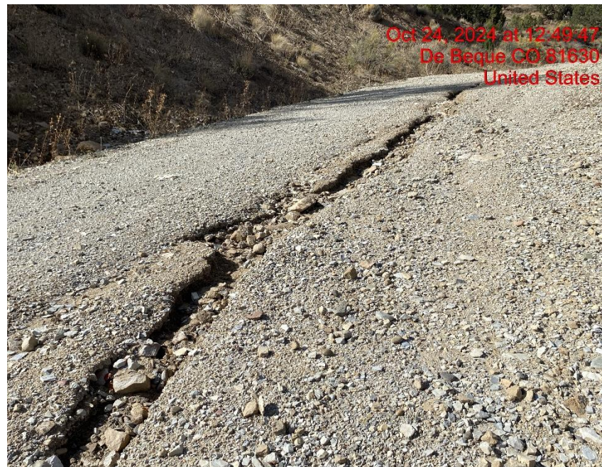
Rill Erosion on Lease Road – Photo #04515
