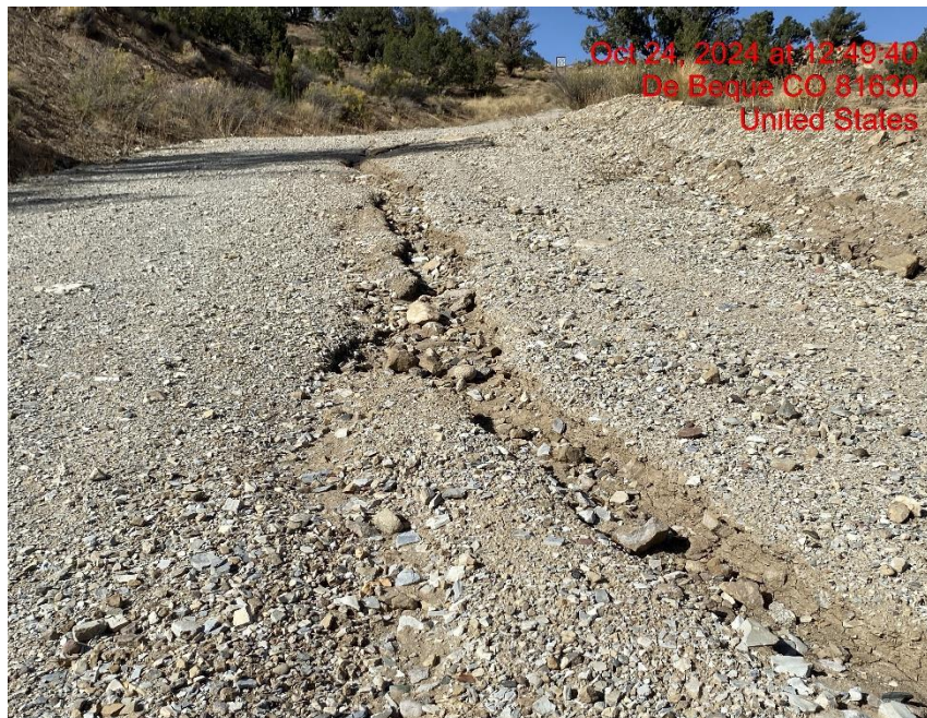
Rill Erosion on Lease Road – Photo #04514
