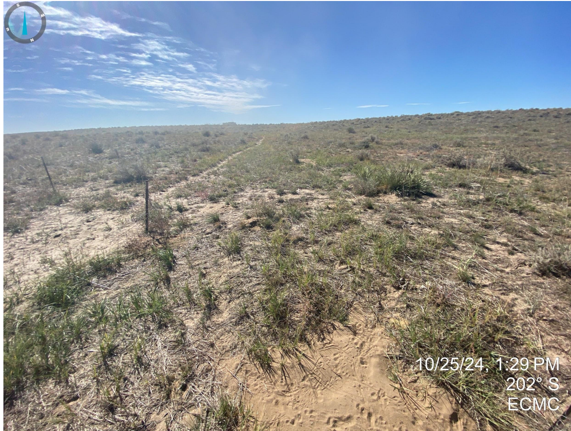
Photo 1. Well markers (t-posts) remain on location and will need to be removed prior to passing final reclamation; therefore, this location will remain "In-Process" until all equipment has been removed.
