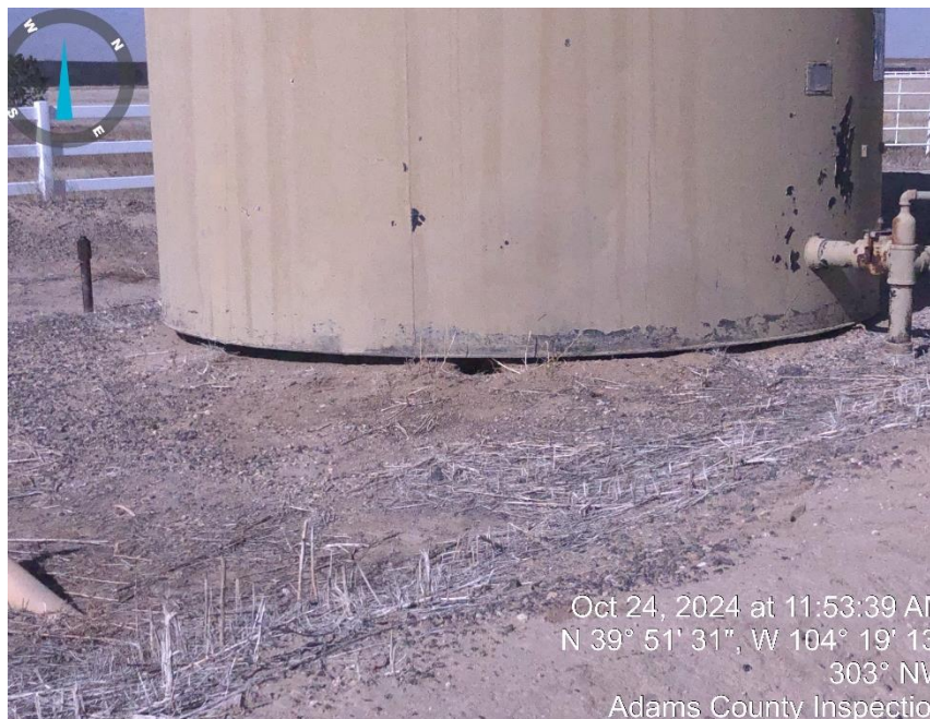
Photo #3 Erosion under condensate tank.
