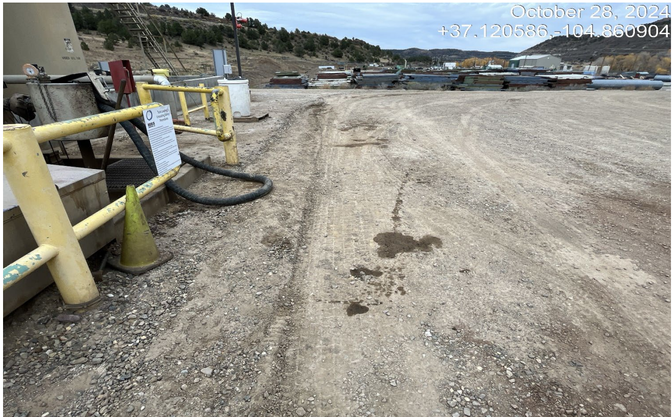
Photo 9. Facing toward the tank battery. There is still oil stained soils where trucks connect to the hoses.
