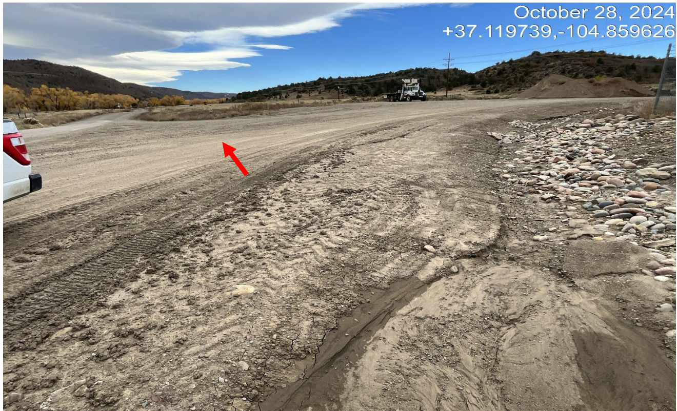
Photo 2. Facing southwest toward the access road adjacent to the main road. BMP's need to be installed to prevent sediment transport onto the road. A berm or track pad or other BMP is needed at the area of red arrow.
