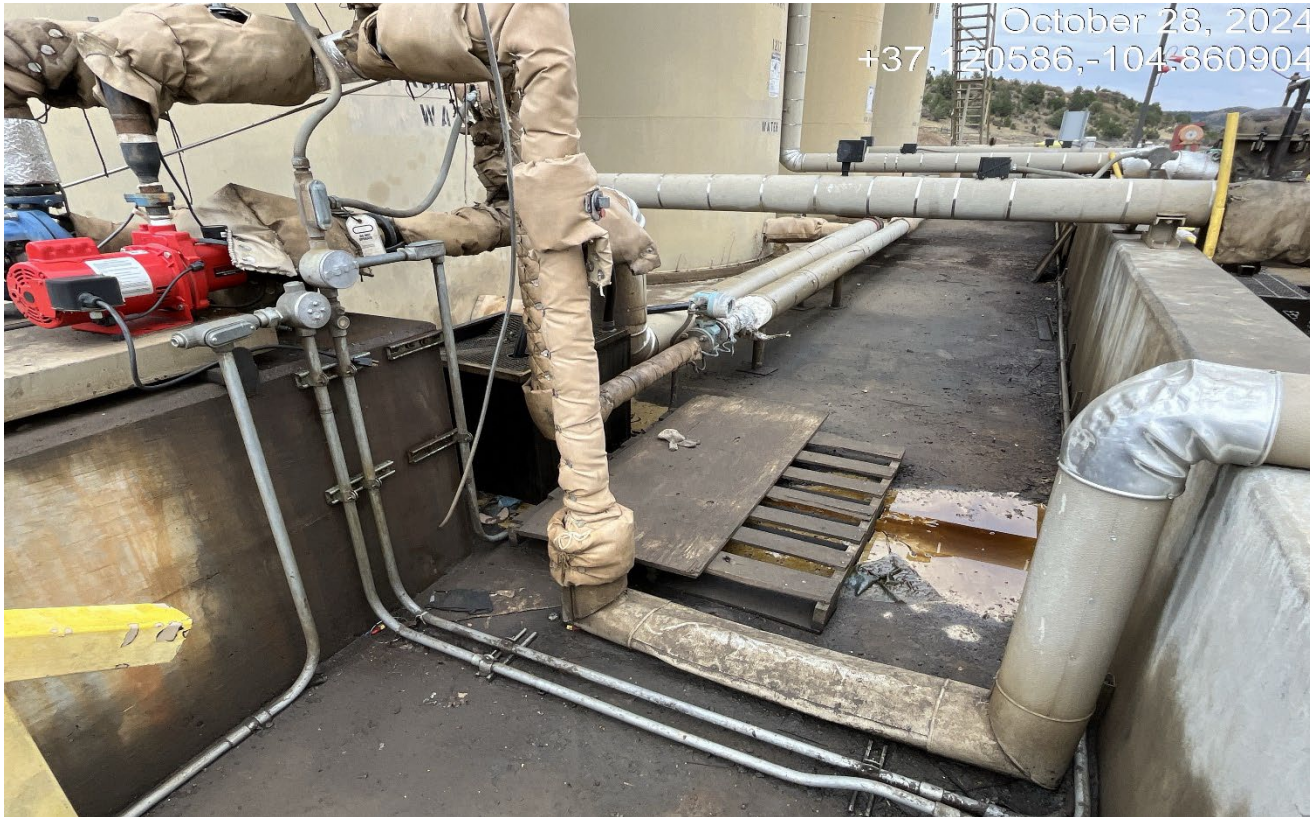
Photo 8. There is oily fluid inside the tank containment area that needs to be cleaned up.
