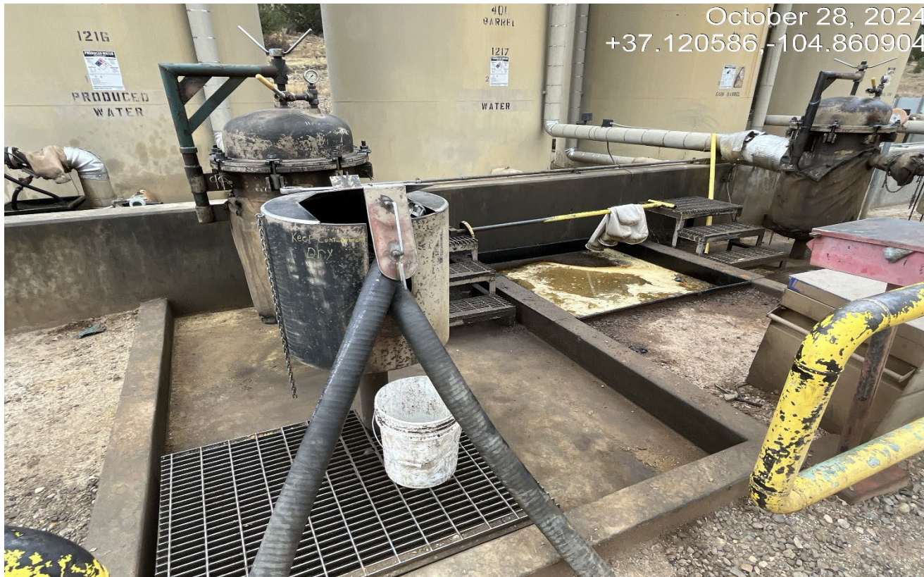
Photo 7. There is oily fluids in the secondary containment. Additionally netting must be installed to prevent wildlife entry. Previous CA was not completed.
