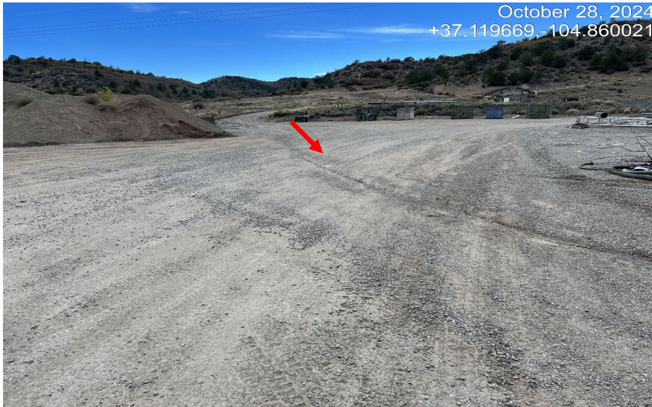
Photo 4. Facing west. It appears stormwater is flowing cross the location contributing to stormwater erosion in previous photos.
