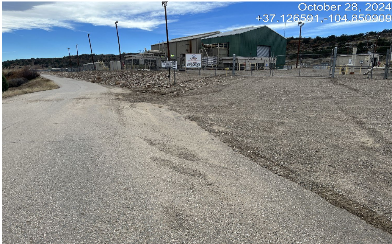
Photo 1. Facing southwest along the main road to the compressor facility. The road was regraded but additional erosion has since occurred.
