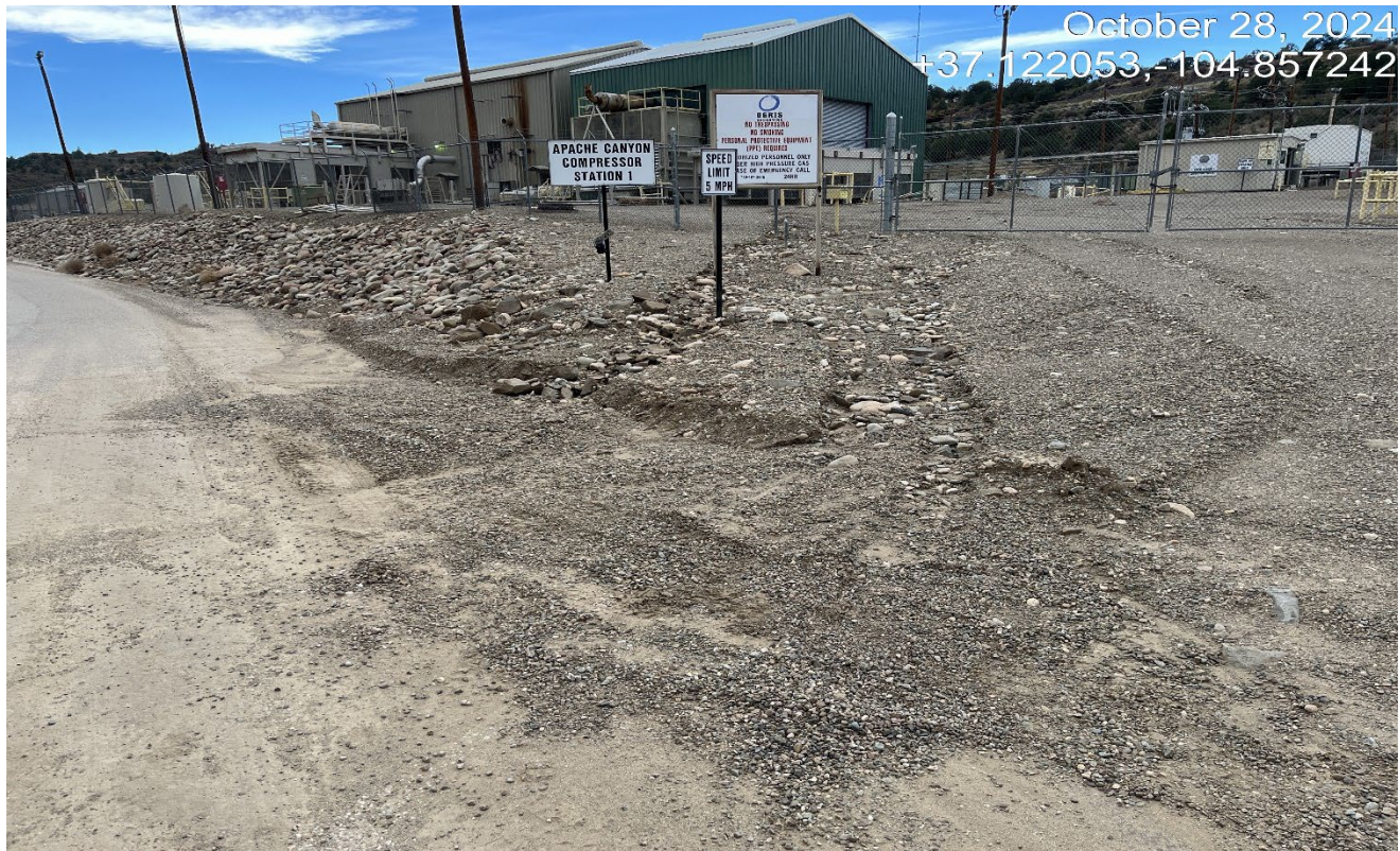
Photo 2. Facing toward the compressor facility. Stormwater erosion is depositing gravel and sediment onto the road. BMP's must be installed to prevent erosion..
