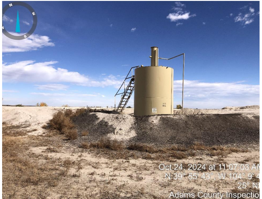
Photo #6 P/W tank, weeds on berm & NFPA placard faded and needs replaced .
