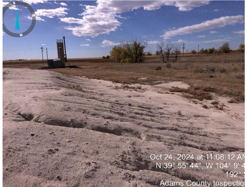
Photo #10 no BMPs in place to prevent berm sediment from leaving location.
