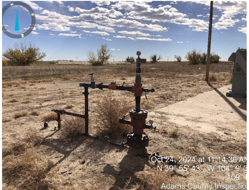
Photo #14 Well head, no sign on well head & weeds around well head.
