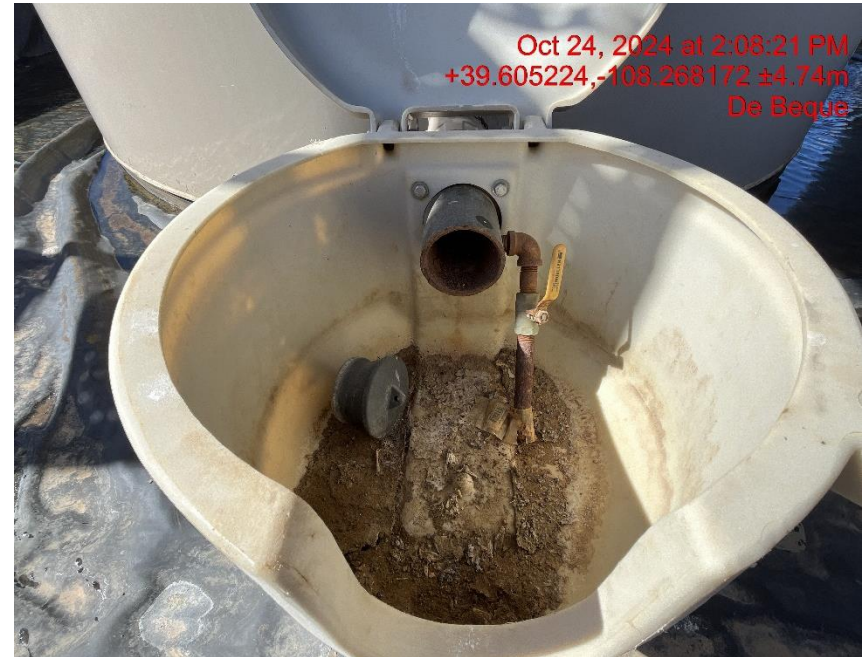
Photo # 8023 Open ended load line
